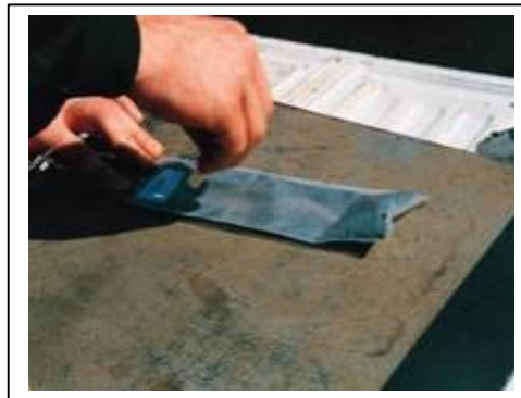
100 grams of Galvpatch being mixed for site repairs of hot dip galvanized steel
