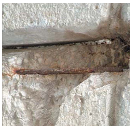
Figure 9: Repairs to the concrete on this bridge structure proved to be unsuccessful in that the corroding reinforcing bars have again removed the concrete.
