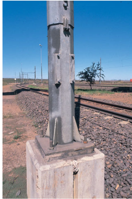
Figure 2 (above) and Figure 3 (above right): Corrosion protection of holding down bolts should be equal to that provided for main structures.
