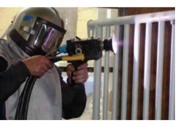
method are required. Upon contact, the particles flatten onto the surface, freeze and mechanically bond, firstly onto the roughened substrate and then onto each other as the coating thickness is increased. In thermal spraying flamespray and arcspray are normally used for finishing coatings.
