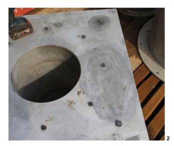
**1** Bearing plate: A typical bearing plate with bolts and some refurbished areas. Note the colour variation as the hot dip galvanizing coating weathers from a light to dull grey patina.
