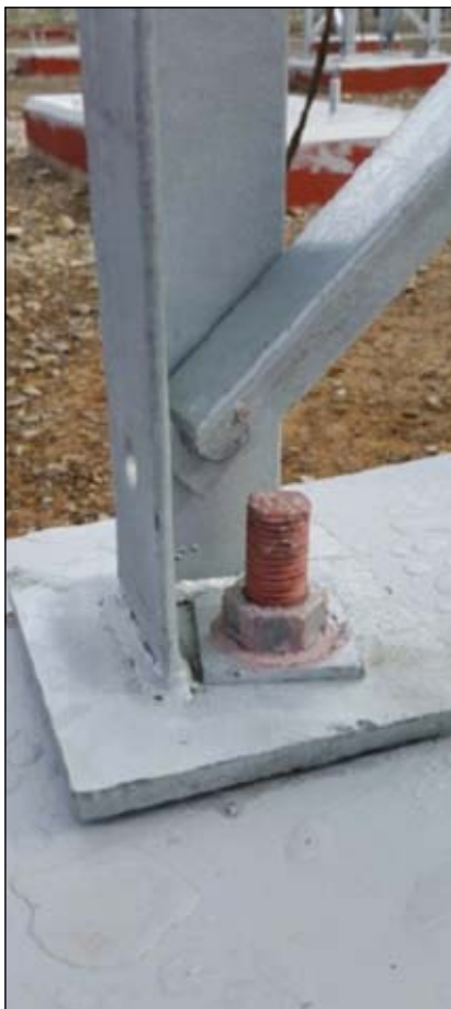
Newly Hydrophobic HRSCA coated substation foundations.
