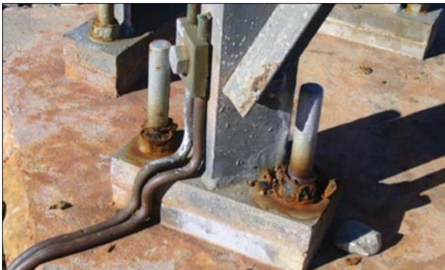
Corroding anchor bolts and nuts.
