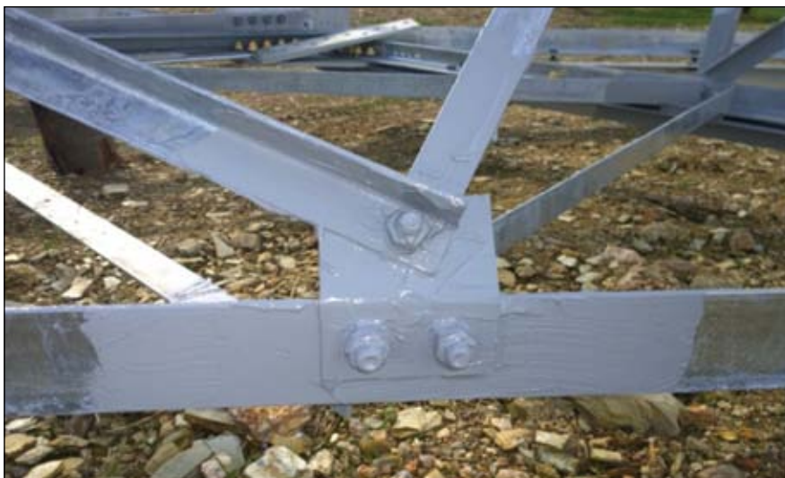
HRSCA used as an active joint sealing technology over hot dip galvanized components and fasteners.
