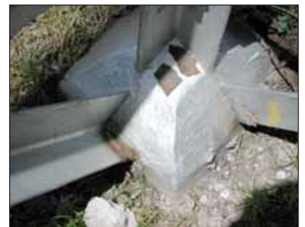
Prevention against differential aeration after erection may not have the desired long term benefit.
