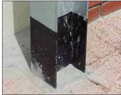
A paint film extending some 200 – 300mm above and below the ground level will prevent differential aeration.
