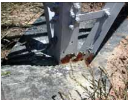
Less effective prevention of differential aeration.
