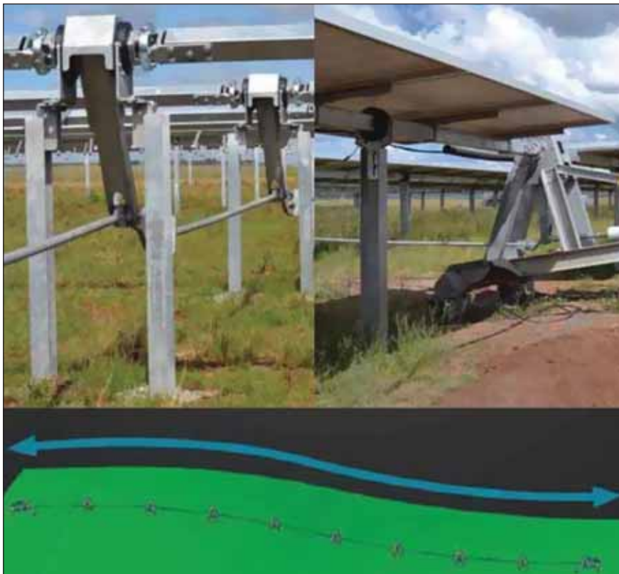
Figure 6: System allowing for solar tracking with terrain irregularities. Galvanized steel rotating supports (10) .
