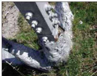
Prevention against differential aeration after erection may not have the desired long term benefit.
