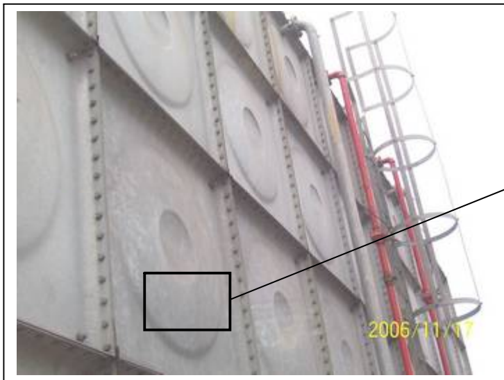
Weathered hot dip galvanized surface finish, dull matt grey
