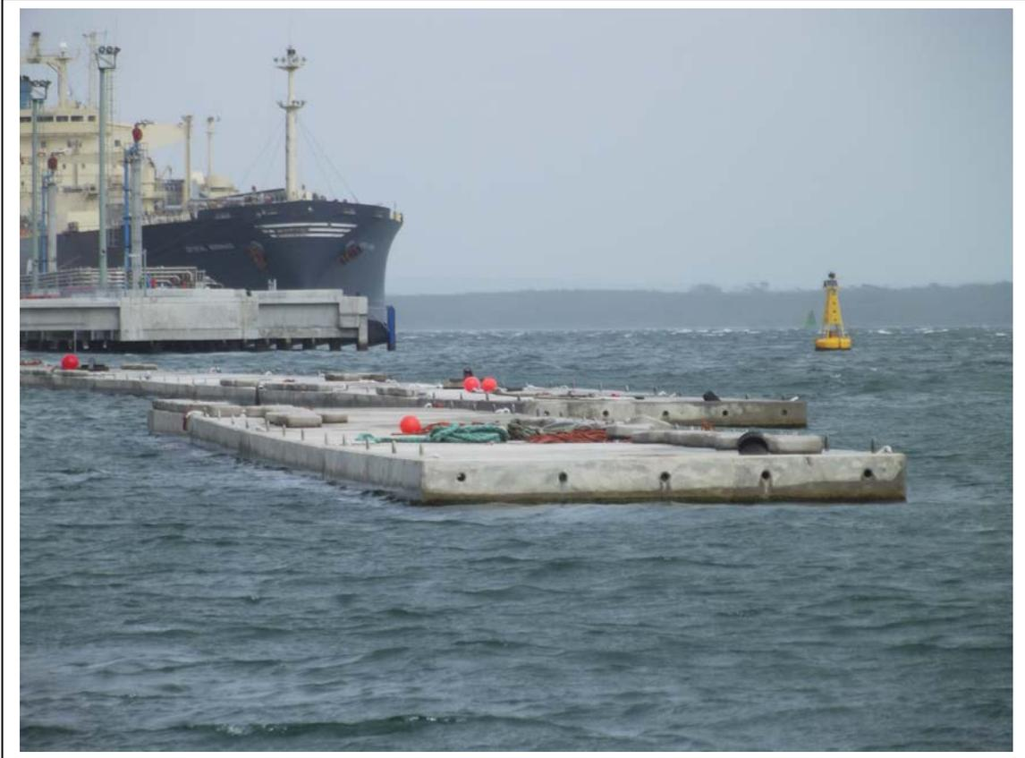
**Hot dip galvanized reinforcement in cast concrete pontoons being floated out in preparation for positioning and anchoring to the sea bed**
