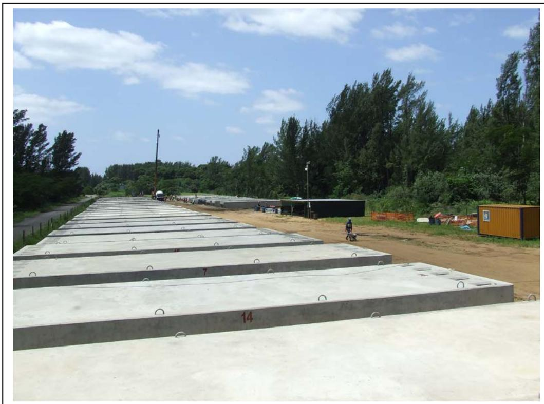
**Completed Concrete Pontoons waiting installation**
