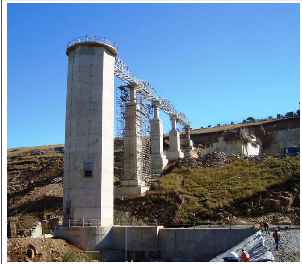
M1150 Ludeke Dam – Pedestrian Steel Bridge Eastern Cape
