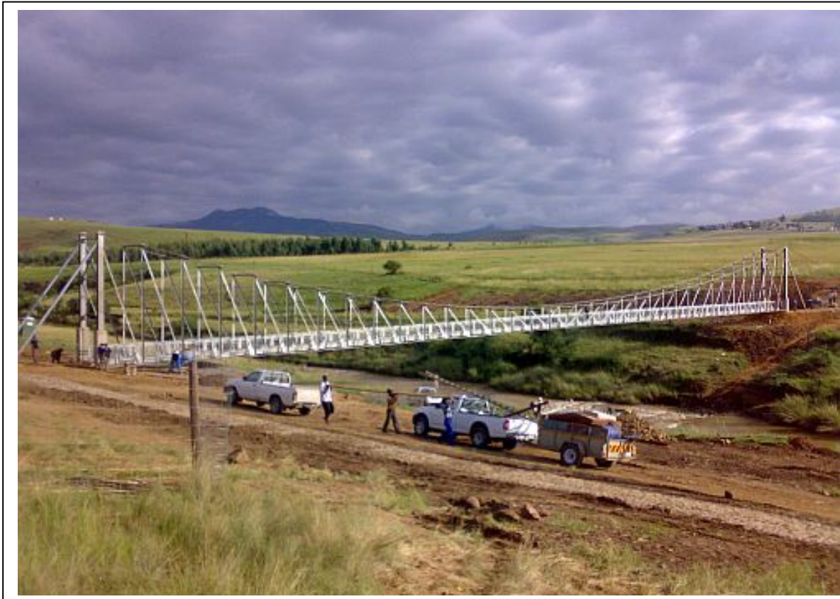
Bisi Pedestrian Bridge Kwazulu Natal Umzimkhulu
