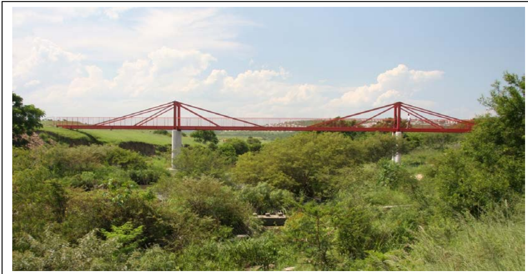
Zwelitsha Pedestrian Bridge over the Buffalo River Eastern Cape Hot Dip Galvanized and painted
