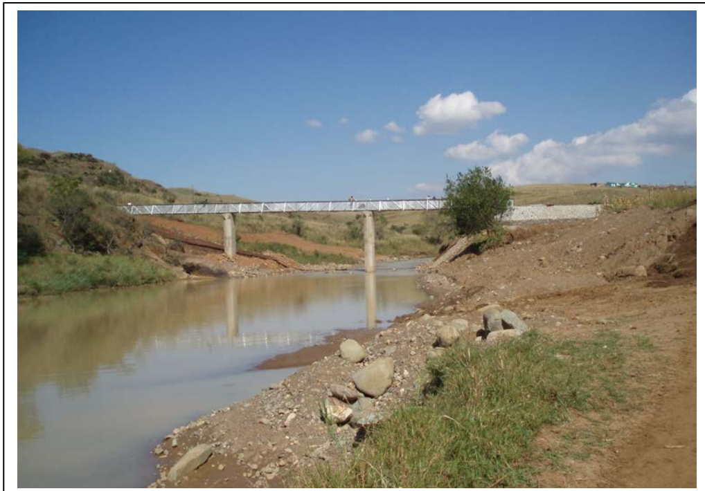
Insuze Bridge - Kwazulu Natal
