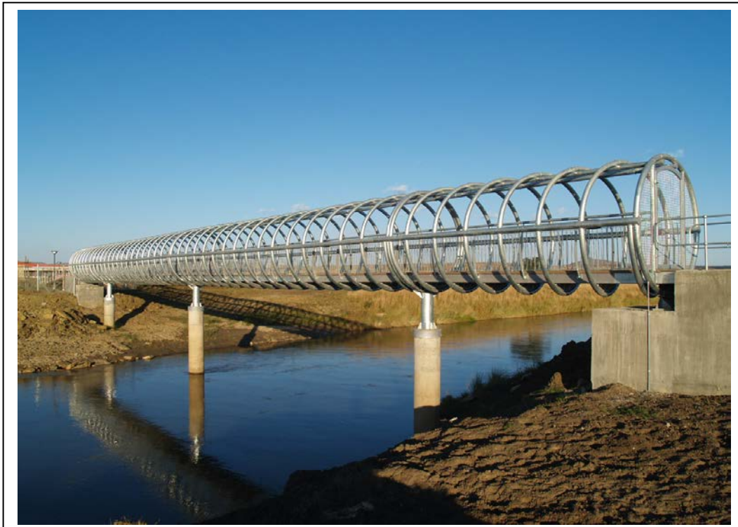
Ncome Museum Pedestrian Spiral Bridge Kwazulu Natal – the site of the Battle of Blood River 16 December 1838
