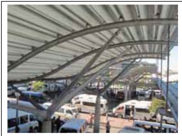
Views of the busy Bellville Transport Interchange showing the curved purlins and 'upside down spider' supports
