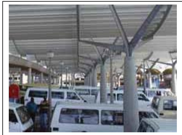
Views of the busy Bellville Transport Interchange showing the curved purlins and 'upside down spider' supports
