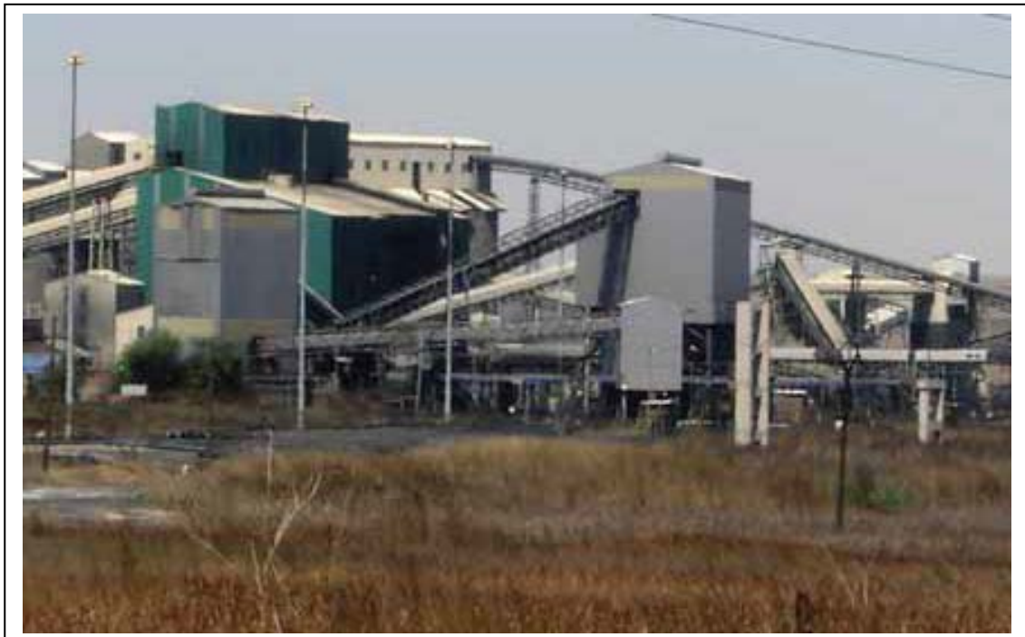
General view of Douglas Colliery
