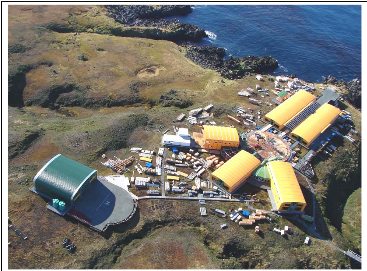
An aerial view of the base under construction
