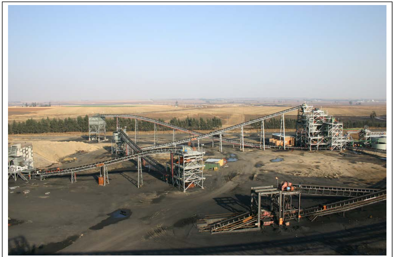
General view of the extensions at the Leeupan colliery
