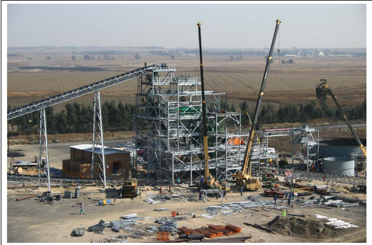
Part of the new plant under construction
