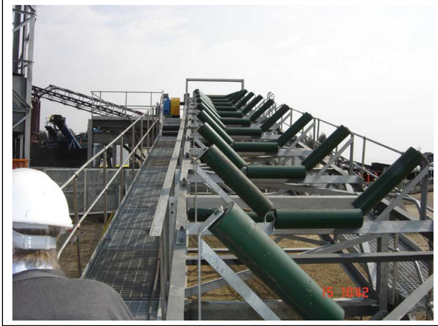
Associated coal conveyor system under construction
