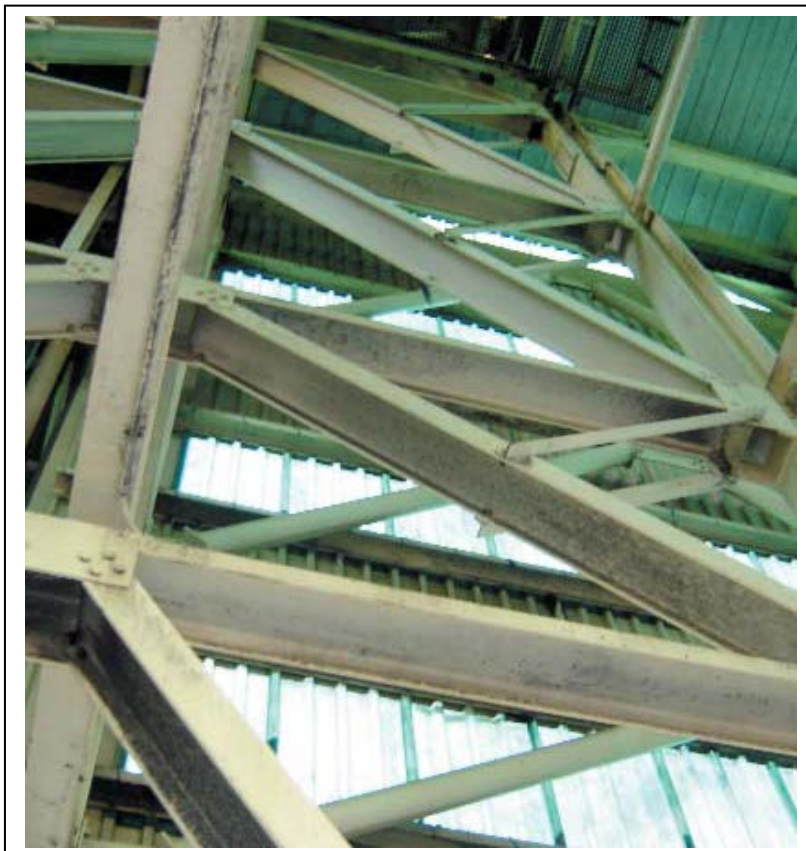
General view of the structure at Goedehoop Colliery in 2005
