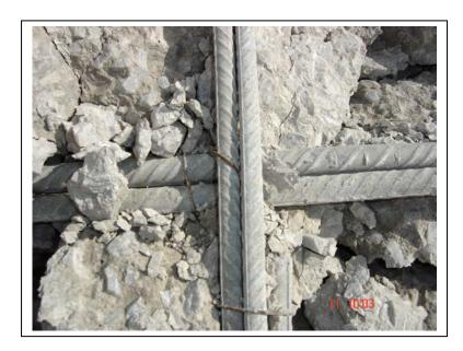
The condition of exposed hot dip galvanized reinforcement found during the demolition of the 40 year old bridge was, with isolated exceptions, found to be exceptional condition
