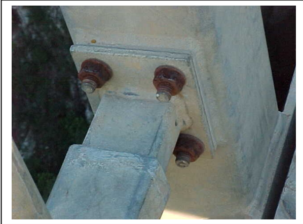
Electro-plated fasteners that have corroded due to insufficient zinc coating thickness
