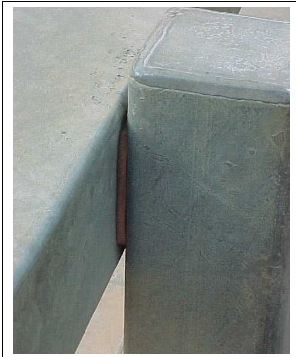
Electro-plated fasteners that have corroded due to insufficient zinc coating thickness
