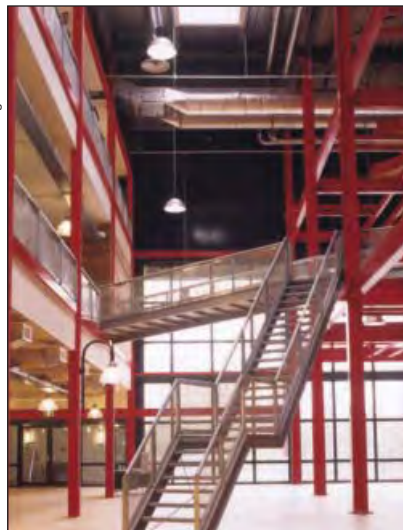
Interior steelwork of an industrial company.
