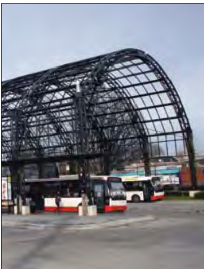
Open structure over bus terminal at Heerlen railway station.
