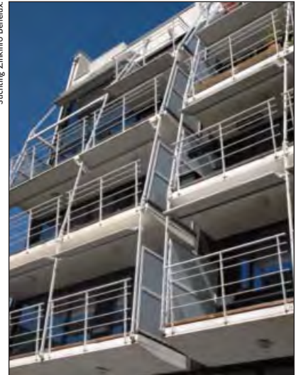
Luxurious apartments in Brussels incorporating balconies hanging from the roof (winner Benelux Trophy- Hot Dip Galvanizing 1997).
