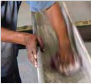
Duram duplex coating surface preparation: detergent wash and water rinse.
