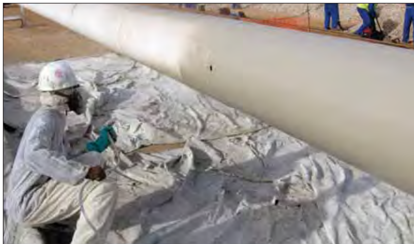
Light masts being painted on site.
