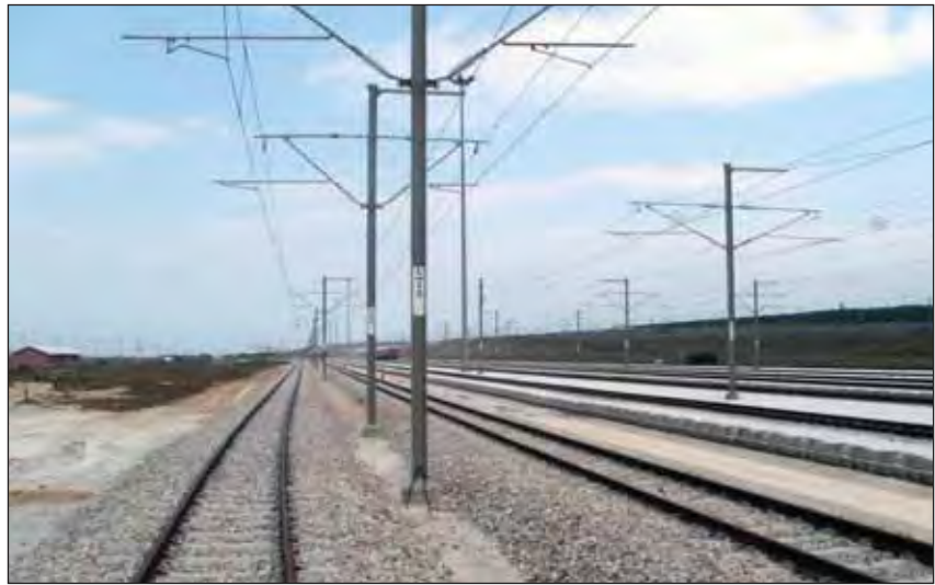
A general view of the duplex coated masts.
