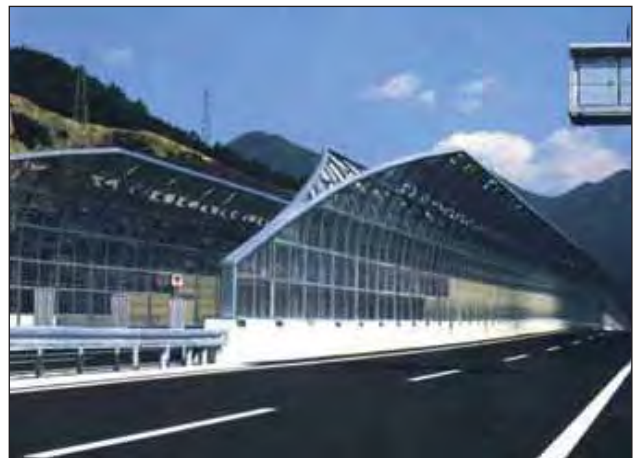
Soundproof walls for Hiroshima-Iwakuni Highway.
