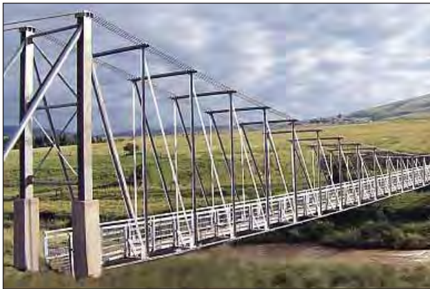
Bisi Pedestrian Bridge.
