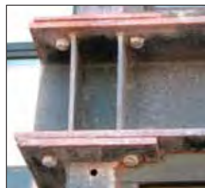
Duplex coating systems have failed near the coast due to inadequate substrate preparation or an inappropriate paint system.
