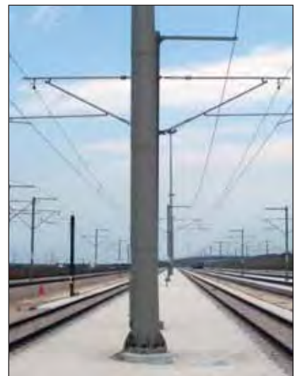
Foundation joints sealed.
