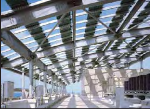
Solar panel shelter and louver of local government office building (above left and right).
