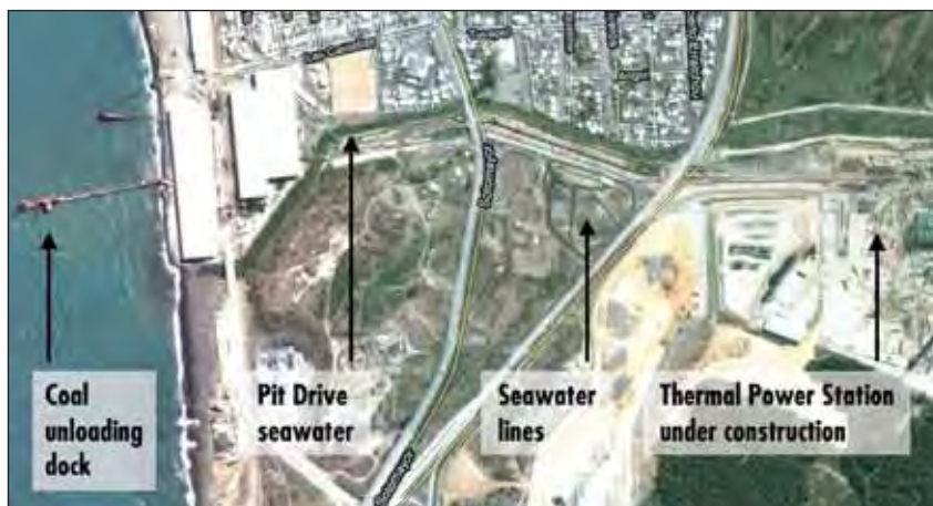
Overview of the construction of the Colbún's thermoelectric plant in Coronel showing the coal loading dock, sea water lines and the construction zone of the plant.
