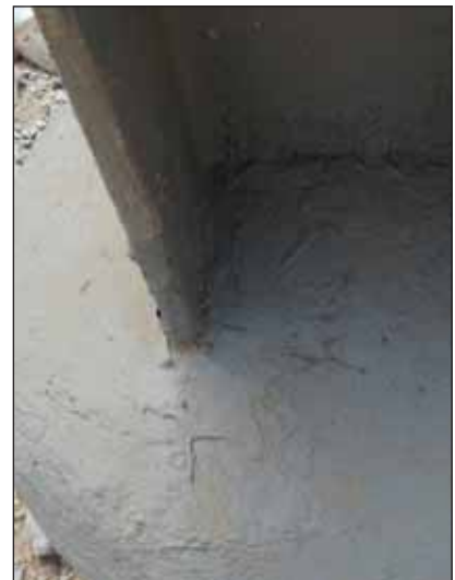
Foundation joints sealed.
