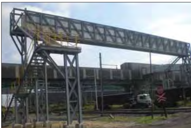
Transnet Pedestrian Bridges.
