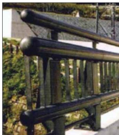
Hand rail (galvanized and chemical treatment).
