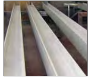
Prime coat: acrylic primer with anti-corrosion pigment.
