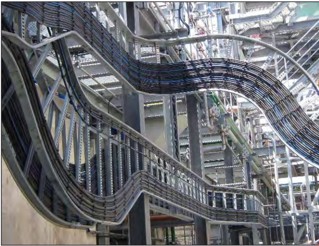
Two views of edge mounted cable ladders for a recent major project.
