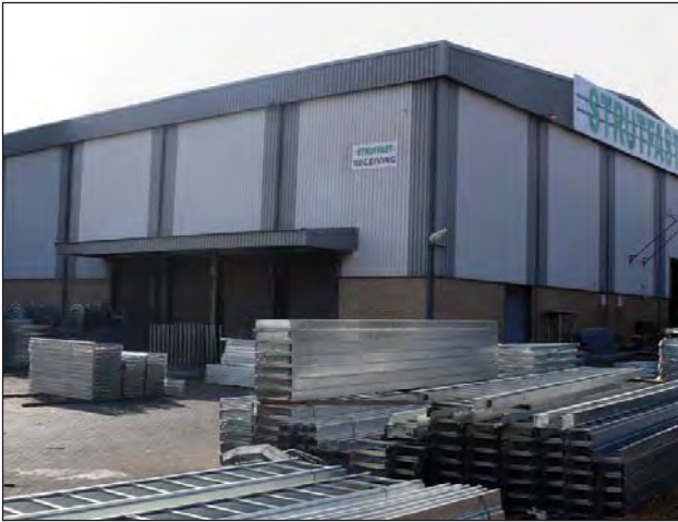
A view of external and internal storage facilities at Strutfast.
