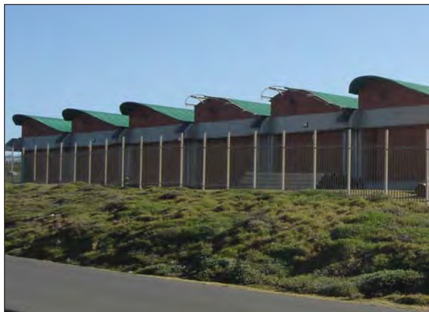
General view of the building.
