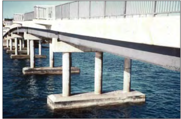
The new Watford Bridge (1979) reinforced with galvanized rebar.
