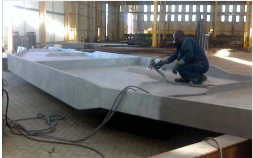
Thermal metal spraying in the workshop.
