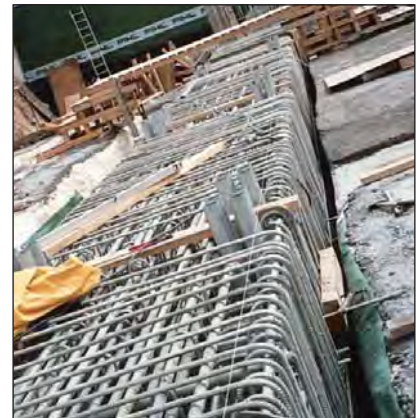
Waste treatment facility, Bermuda.
