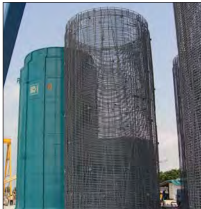
Outfall pipes, Singapore.
