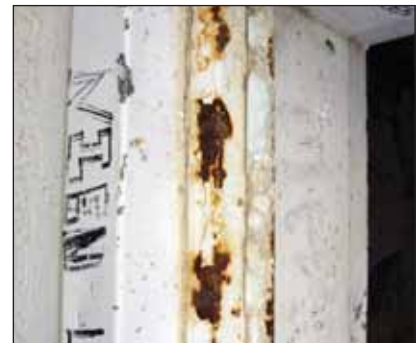
Window 1 on which an evaluation was carried out (left). Close up photo of coating damage and subsequent corrosion (right).
