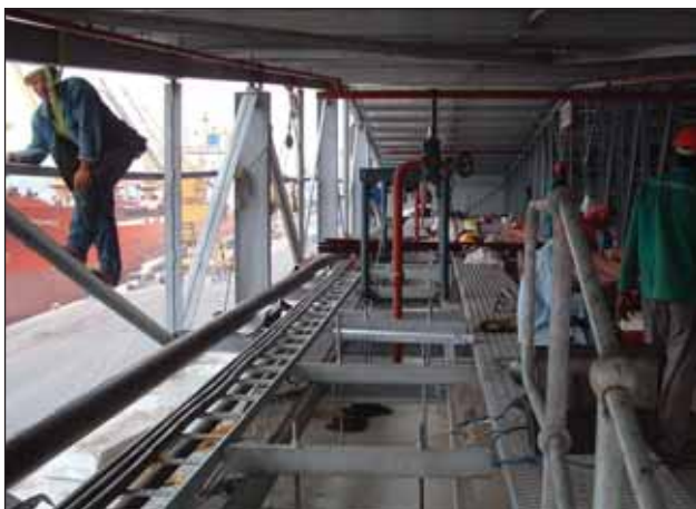
Much of the steelwork in the storage terminal was hot dip galvanized.
