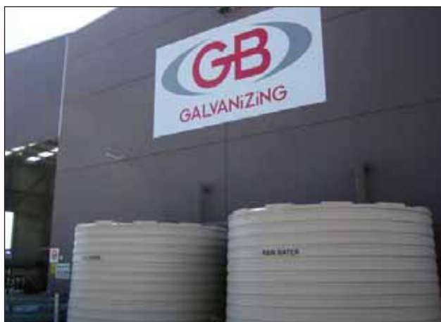
Rain water off the building is stored in these tanks for subsequent use in the process.
