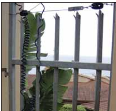
The pedestrian gate was installed in 2004 (left) and from coating thickness readings (right) the coating was hardly affected and in good condition. There were no signs of surface zinc chloride on the coating.
