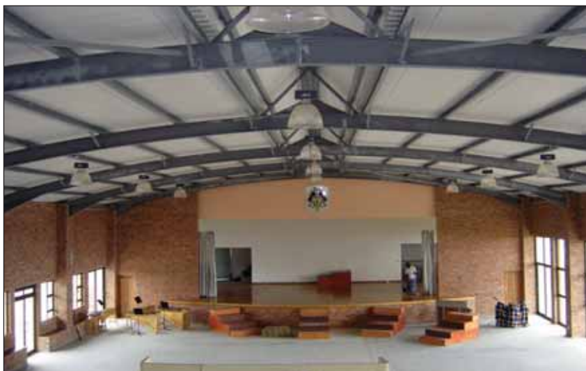
Hot dip galvanizing was used to protect the structural steel supporting the roof cladding.
