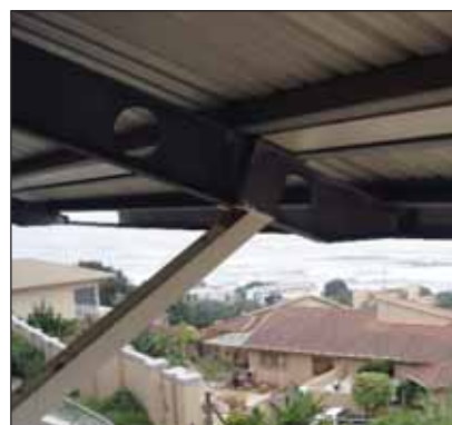
Photo left, showing the eaves from upstairs on the landward side and photo right, the eaves on the seaward side, indicating the different micro-climatical conditions that the hot dip galvanized coating is subjected to.
