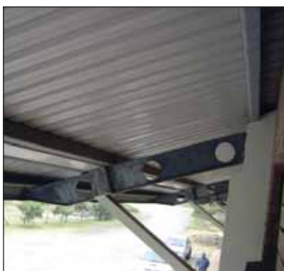
Photo left, showing the eaves from upstairs on the landward side and photo right, the eaves on the seaward side, indicating the different micro-climatical conditions that the hot dip galvanized coating is subjected to.
