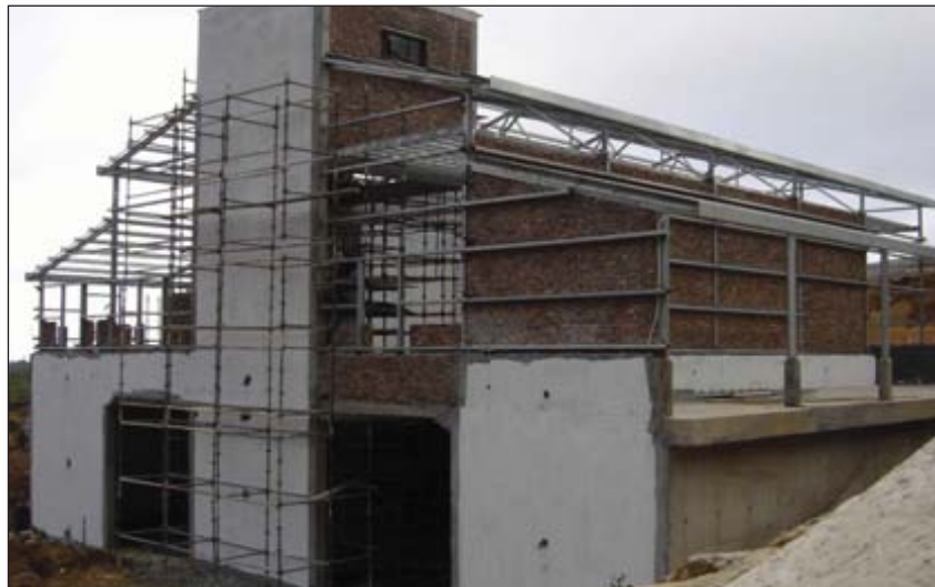
All structural steelwork was hot dip galvanized with the veranda columns left unpainted. This was done in order to monitor the performance of the hot dip galvanized coating over the ensuing years.
