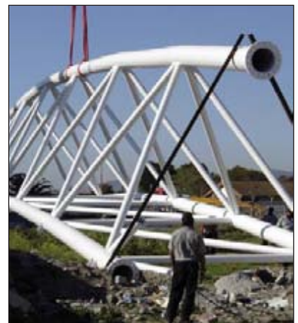
End view of a completed section about to be lifted into position on site.
