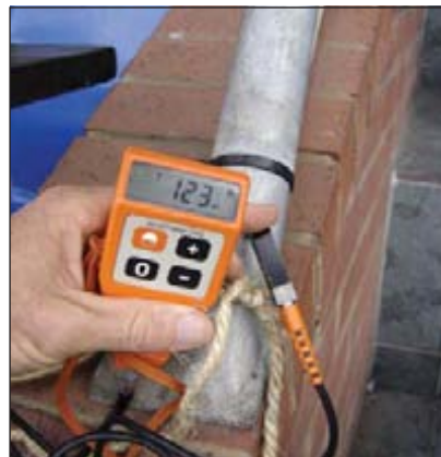
Typical coating thickness on the handrail.
