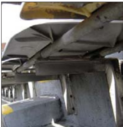
The hot dip galvanized seat brackets.
