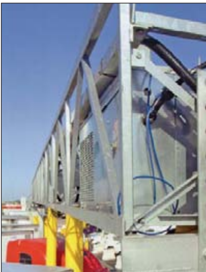
Advanced Truckstop Electrification Terminal (ATE).
