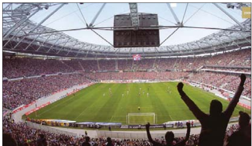
The large cube in the centre of the Frankfurt's Waldstadion, the steel of which was largely hot dip galvanized, often interfered with the camera's view.
