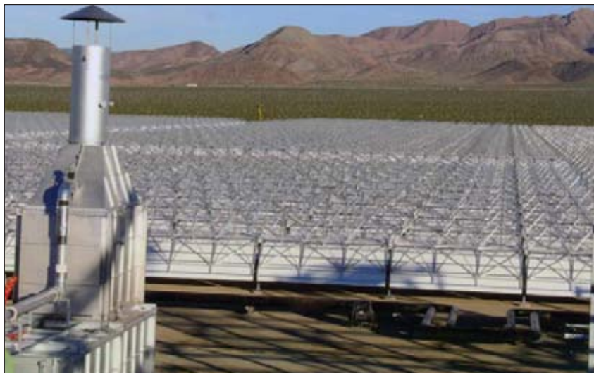
Nevada Solar One Solargenix Energy.
