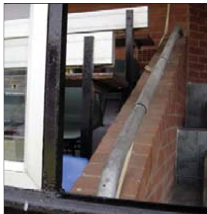
The unpainted hot dip galvanized handrail at the press box.
