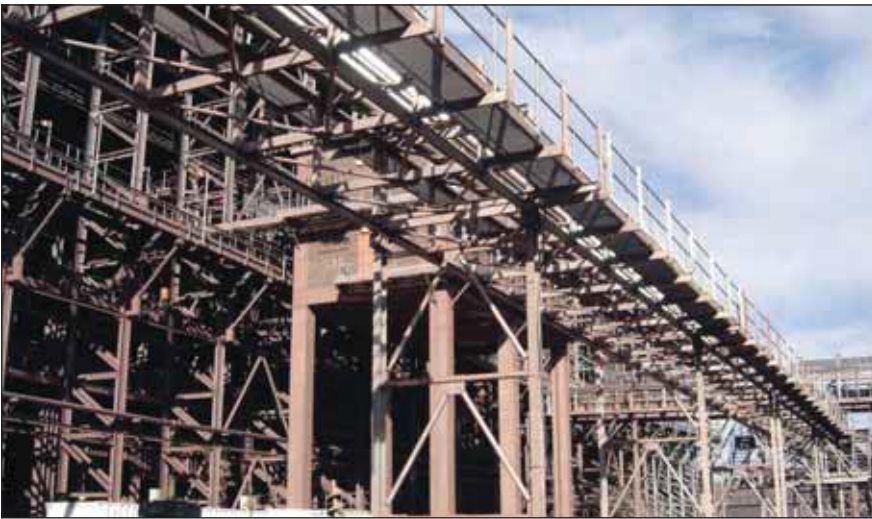
Photos 24 – 27 show the Sishen expansion project including some 22 000 tons of hot dip galvanizing in the form of process and conveyor steelwork.
