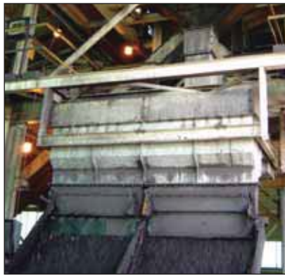
Photo 20: The coal washing plant.
