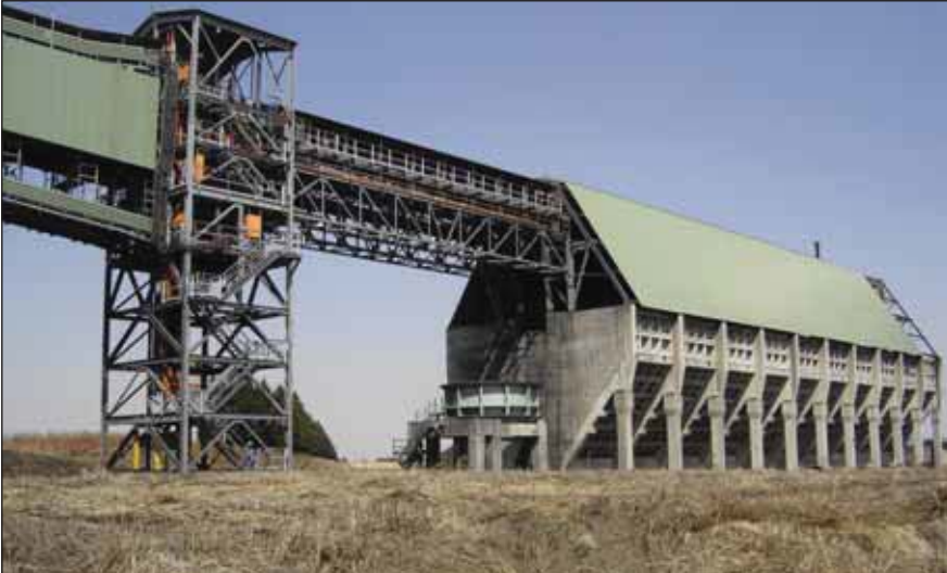
Photos 13 – 17 (from top left clockwise) show views of the conveyors of Isibonella Colliery; the transfer tower; another view of a long conveyor and the transfer tower and hopper.
