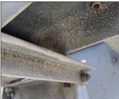
Coating contaminants removed and residual coating thickness measured 180 and 148µm respectively.
