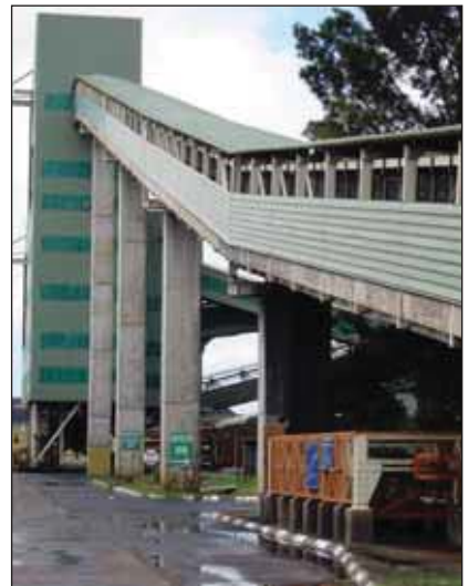
Photo 19: The transfer tower.
