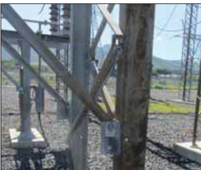
Discolored hot dip galvanized coating including coating thicknesses of 376 and 338µm respectively.
