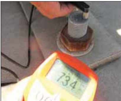
Holding down bolt coating thickness 73.4µm.
