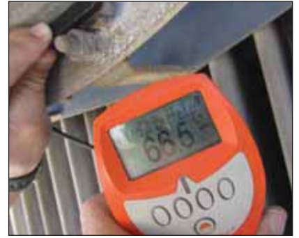
Coating thickness measured 66.5µm.
