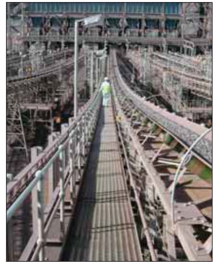
Photos 24 – 27 show the Sishen expansion project including some 22 000 tons of hot dip galvanizing in the form of process and conveyor steelwork.
