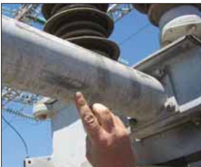
Hot dip galvanized tube cleaned of contaminants and coating thickness readings taken as 106 and 133µm respectively.
