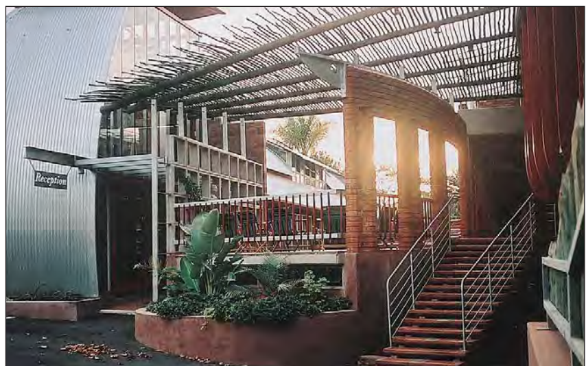
The north and south wing run parallel to each other and enclose a cloistered garden that terminates in a covered patio centre. The main dining room is on the right and the reception offices on the left. Note the timber banisters used to connect the hot dip galvanized steel hand rails (photo taken in 2001).
