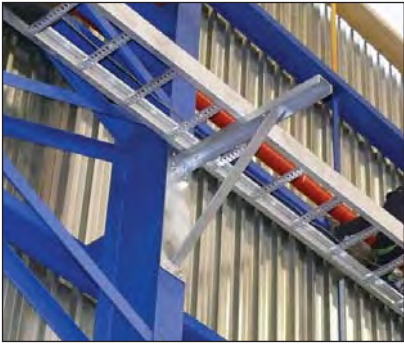
Trident using Strutfast's LONGBOW 20B Cable Support System, which has been designed and developed by Strutfast in compliance with the NEMA Standard VE-1. The Class Designation 20B signifies that it is capable of carrying a cable working load of 112kg/m over an unsupported span of 6 metres. The heavy duty supports were also designed and supplied by Strutfast. (All items hot dip galvanized to ISO 1461 by Galvadip).
