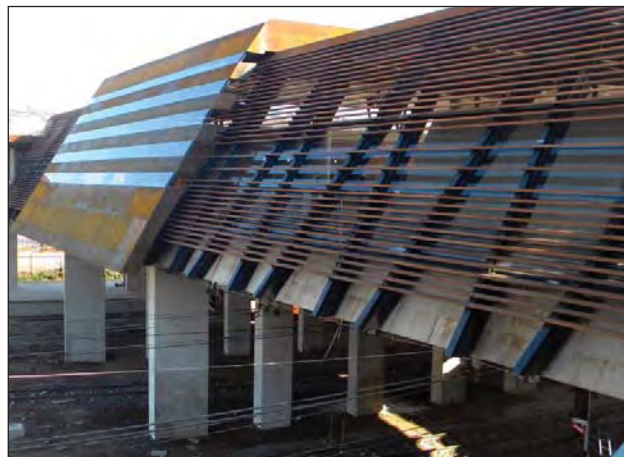
One of the views showing the use of Corten Material fixed to a duplex coated frame.
