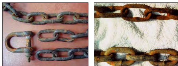
Figure 1 (photo above left). The re-galvanized 8mm hot dip galvanized mooring chain after 14 years service in the Vaal Dam. The links of chain in the middle of the photograph were the worst corroded – this end had been attached to the Dee-shackle below the mooring buoy where it experienced the greatest amount of grinding. The links at the bottom had been above water much of the time (attached to the boat) and the links shown at the top represent the average condition the rest of the chain. Figure 2 (photo above right). The chain as it appeared in 1998.
