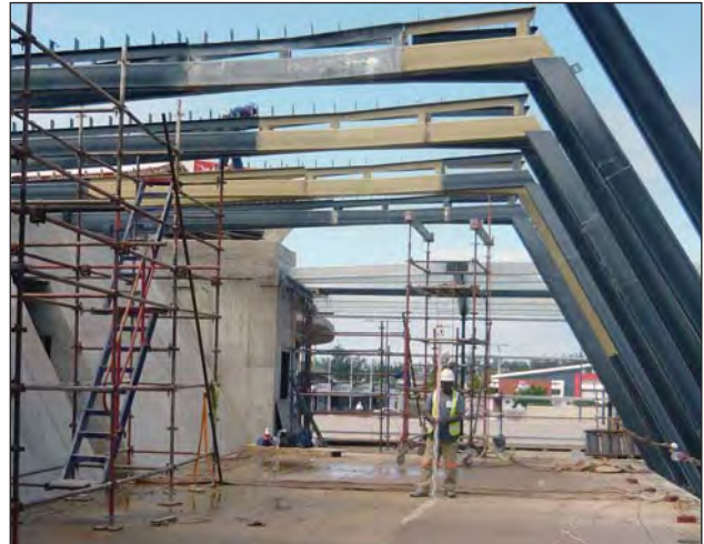
Hot dip galvanized steel in the process of being painted.
