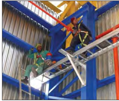
Trident using Strutfast's LONGBOW 20B Cable Support System, which has been designed and developed by Strutfast in compliance with the NEMA Standard VE-1. The Class Designation 20B signifies that it is capable of carrying a cable working load of 112kg/m over an unsupported span of 6 metres. The heavy duty supports were also designed and supplied by Strutfast. (All items hot dip galvanized to ISO 1461 by Galvadip).
