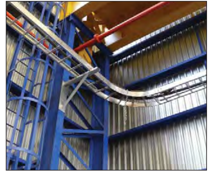
Trident using Strutfast's LONGBOW 20B Cable Support System, which has been designed and developed by Strutfast in compliance with the NEMA Standard VE-1. The Class Designation 20B signifies that it is capable of carrying a cable working load of 112kg/m over an unsupported span of 6 metres. The heavy duty supports were also designed and supplied by Strutfast. (All items hot dip galvanized to ISO 1461 by Galvadip).
