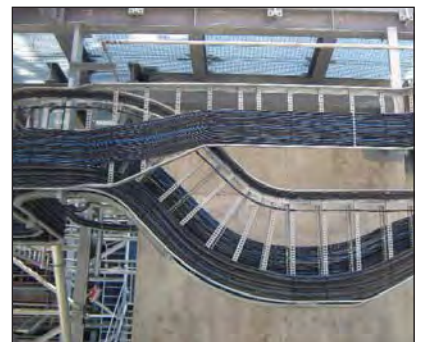
The Strutfast product used on this installation is our SB75 STRONGBOW Cable Ladder. The finish is hot-dip galvanized to ISO 1461 by Galvadip. The installation Contractor is Craig Miller Technical Services.
