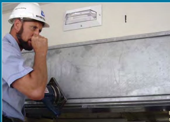
The circular motion of the orbital sander is mild enough to not remove a significant portion of the coating but sufficient to improve the appearance!
