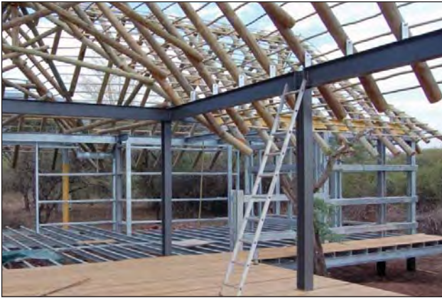
All the sub frames, floor supports and purlins were hot dip galvanized.
