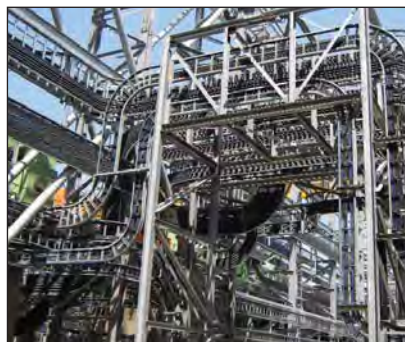
The Strutfast product used on this installation is our SB75 STRONGBOW Cable Ladder. The finish is hot-dip galvanized to ISO 1461 by Galvadip. The installation Contractor is Craig Miller Technical Services.
