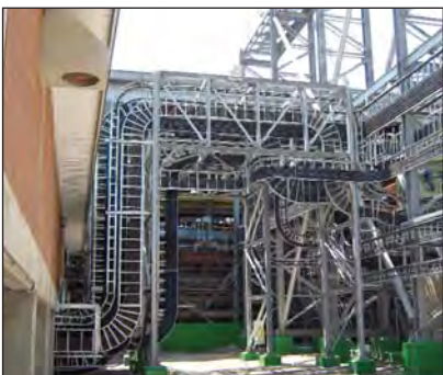
The Strutfast product used on this installation is our SB75 STRONGBOW Cable Ladder. The finish is hot-dip galvanized to ISO 1461 by Galvadip. The installation Contractor is Craig Miller Technical Services.
