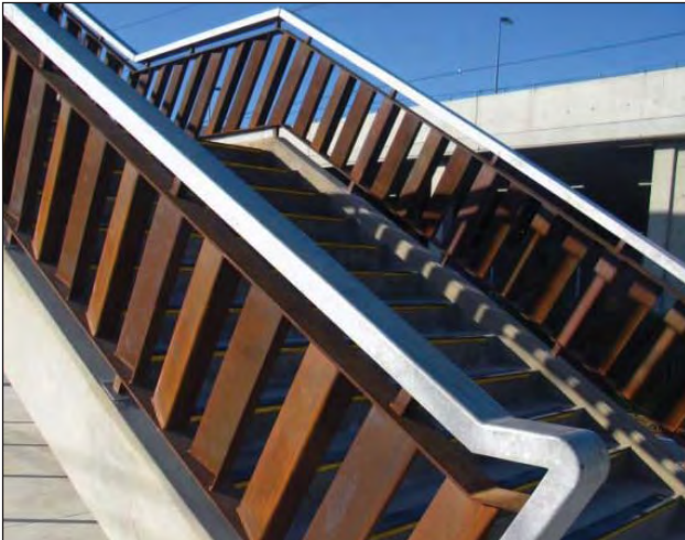
Hot dip galvanized handrailing supported by Corten balustrades.
