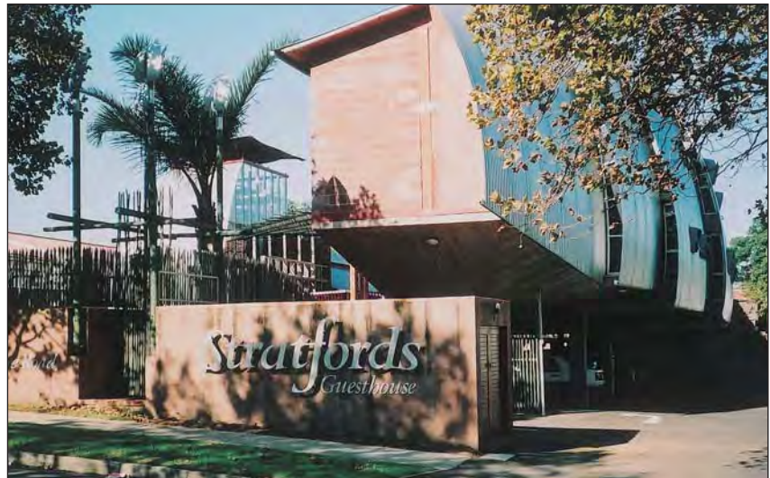
Entrance view showing the front laser cut hot dip galvanized signage, which has back lighting for illumination at night (photo taken in 2001).
