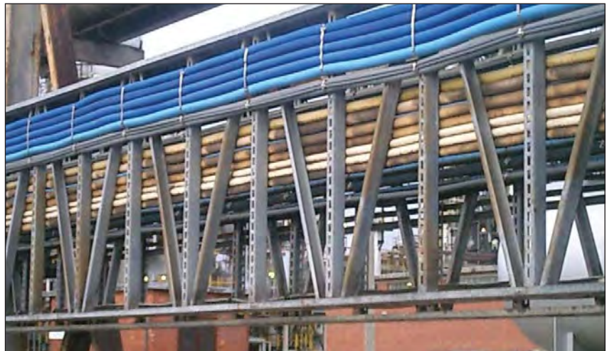
Double sided cable ladder will not easily twist when loaded.
