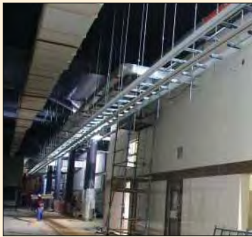
General view of the cable ladders and accessories, were located on site.
