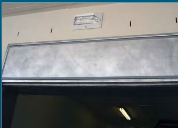
The appearance of the hot dip galvanized coating after using the orbital sander:
