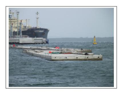
Hot dip galvanized reinforcement in cast concrete pontoons being floated out in preparation for positioning and anchoring to the sea bed
