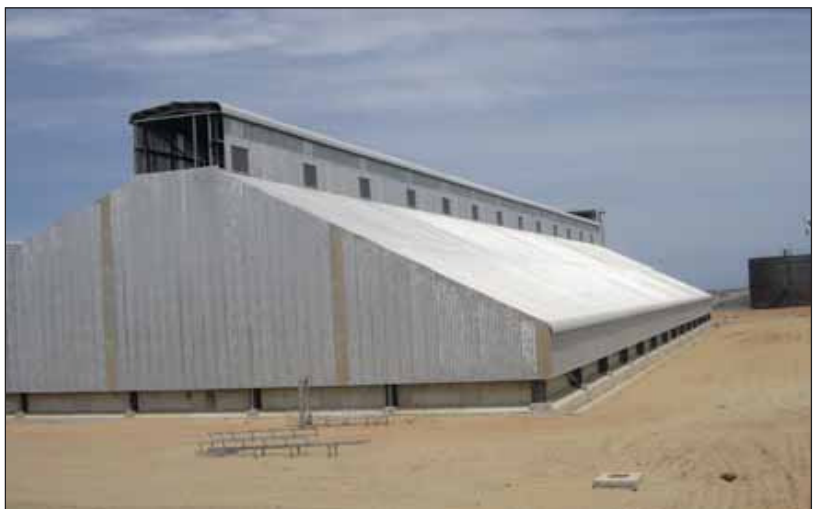
One of three such structures, where refined products will be stored prior to conveyance, via an overland conveyor, to a specially constructed loading pier, for loading onto sea-barges for transhipment to ships anchored offshore
