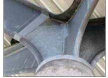
Where Zincfix has been correctly applied there are no signs of premature failure.
