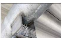
Hot dip galvanized I-Beam tubular purlin support, showing a residual coating thickness of 252µm.
