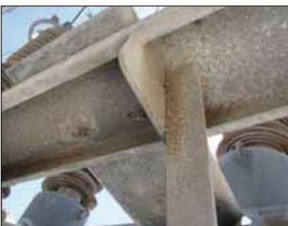
Above left, centre and right: Appearance of the coating on support angle, with residual coating thickness taken at a cleaned area of 169 and 191µm respectively.
