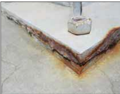
One single base plate showed corrosion on the edge. Residual coating thickness readings of 140 and 165 \mu m were taken adjacent to the corroded area. A possible cause is an original over cleaned edge or use of an acidic grout.
