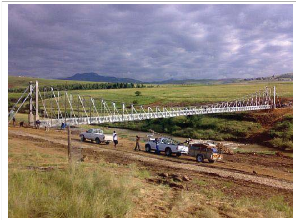
Bisi Pedestrian Bridge Kwazulu Natal, Umzimkhulu
