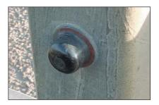
Photo 15. In order to increase the maintenance free life of the main fasteners, plastic covers were introduced, filled with a silicon sealant and then pressed home. Note the insufficiently coated washer (possibly electro-plated), which is now showing signs of corrosion.
