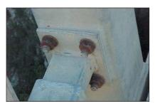
Photo 18. Some fasteners, which were originally inadequately protected require coating repair:
