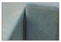
Photo 14. In order to avoid the possibility of crevice corrosion at construction joints, organic washers have been introduced.
