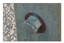
Photo 16 indicates a fastener that has lost its cover and 17 a damaged plastic cover and rusting washer:
