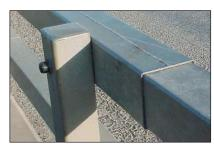
Photos 10 to 13, indicate how slip joint designs can eliminate the requirement for unnecessary site alterations and consequent coating repair:
