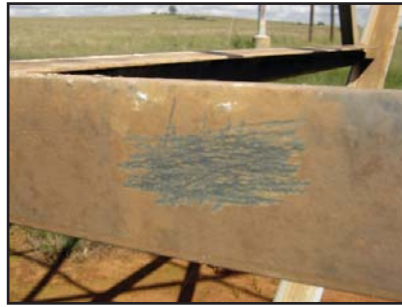
Photos 14 & 15: Site No. 1 – After removing "apparent" rust discolouration, the underlying hot dip galvanized coating measured 65.4µm.
