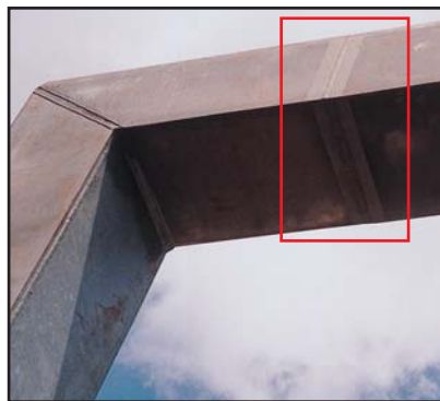
Figure 108. Site welded joint on hot dip galvanized highway sign gantry - repaired by "Zincfix".
