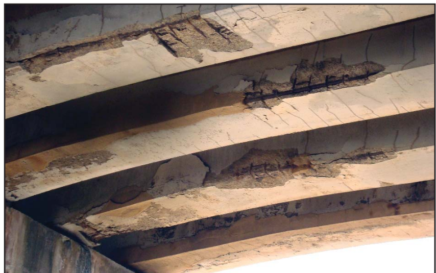
Figure 96. Spalling of the concrete layer on reinforcing steel on the underside of a concrete bridge.
