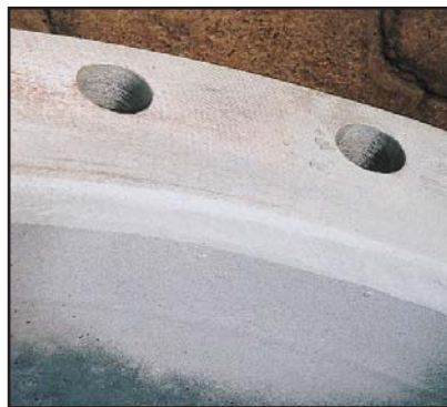
Figure 107. Zinc metal spray applied to a small uncoated area on a pipe section, adjacent to the flange.
