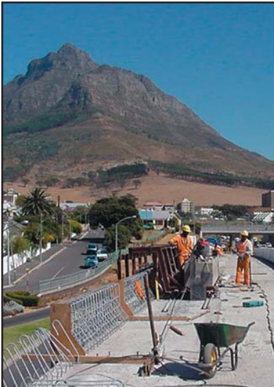
Figure 95. Hot dip galvanized reinforcing bars prior to casting concrete, marine conditions.
