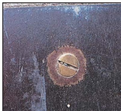
Figure 92. Brass bolt in hot dip galvanized steel on a parking deck.
