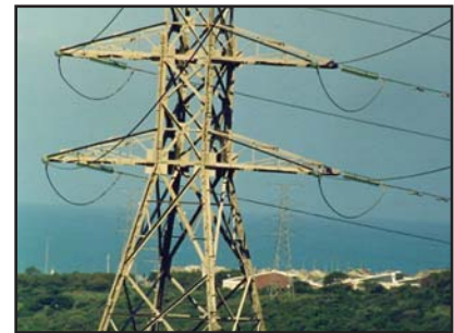
Photo 16: Severe marine coastal conditions. Buffalo-Port Rex Transmission Line situated in East London. At the time of the coating inspection, the towers had been in service for about 25 years.
