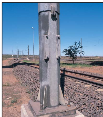
Figures 99 (left) and 100 (right). Corrosion protection of holding down bolts should be equal to that provided for main structures.
