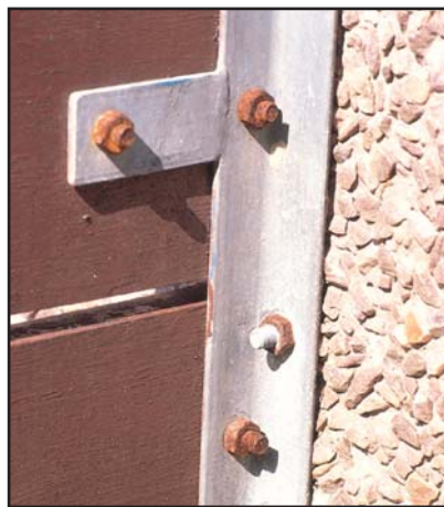
Figure 98. An assortment of zinc coated bolts showing the importance of coating thickness in a particular environment.
