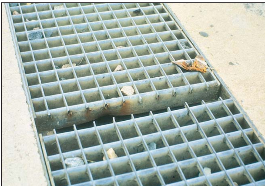
Figure 89. After 20 years of marine exposure, this site cut unrepaired hot dip galvanized steel grating still offers cathodic protection at the cut ends.
