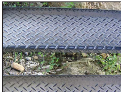
Figure 5. Abrasion resistance of hot dip galvanized vastrap stairs (coating thickness - 49\mu\text{m} , taken 10 years after installation).
