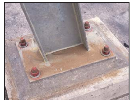
Figures 99 (left) and 100 (right). Corrosion protection of holding down bolts should be equal to that provided for main structures.
