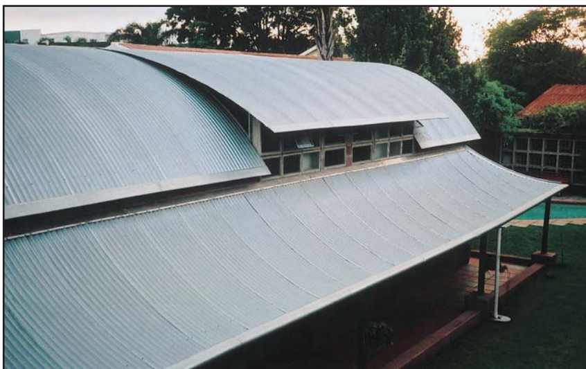
Figure 18. S-Rib galvanized steel sheeting – Z600 coating classification used for architectural applications.
