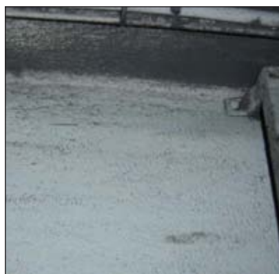
Two examples of the extent and severity of the corrosion conditions on painted steel.
