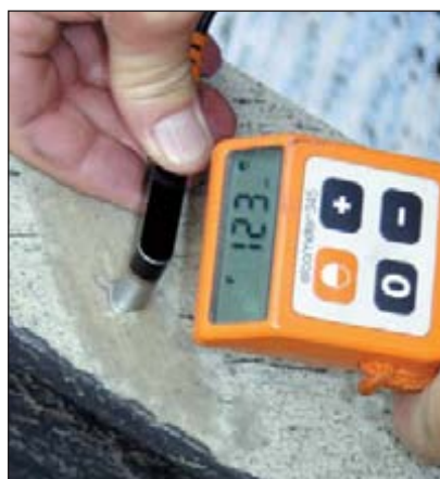
Hot dip galvanized coating thickness (paint removed).
