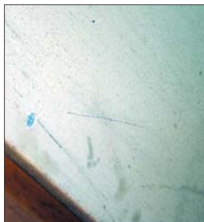
Cross cutting proved that adhesion of the coating was sound.
