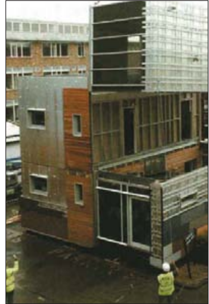
Figure 9. Pre-fabricated room systems being installed in the UK (Materials World, Vol. 13, No. 7, July 2005)
