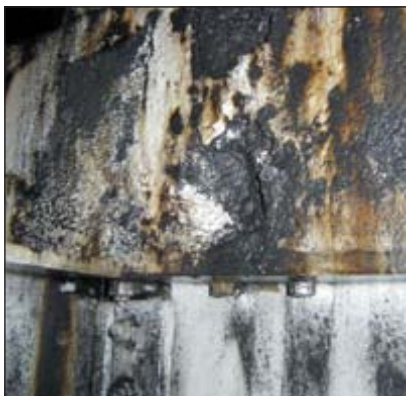
Two examples of the extent and severity of the corrosion conditions on painted steel.
