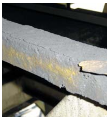
In comparison the paint coating on the carbon steel handrails has failed.
