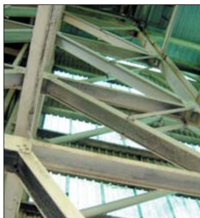
General photo of the structure.
