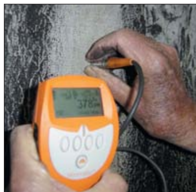
This 378µm coating reading was typical of that found on the structural steel.
