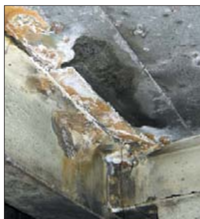
General corrosion conditions of the coal washout facility.
