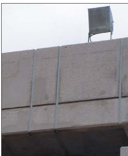
Areas of concrete that have been repaired following the corrosion of the re-bar and the "spalling off" of the concrete. Such repairs are difficult to carry out and generally have limited success.
