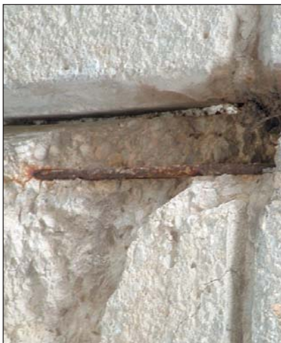
Corroded re-bar resulting in the "spalling off" of the concrete cover:
