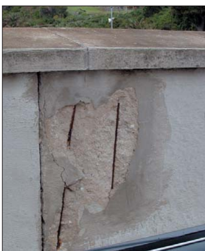
Repairs to the re-bar on this bridge structure proved to be unsuccessful in that the corroding reinforcing bars have again removed the concrete.
