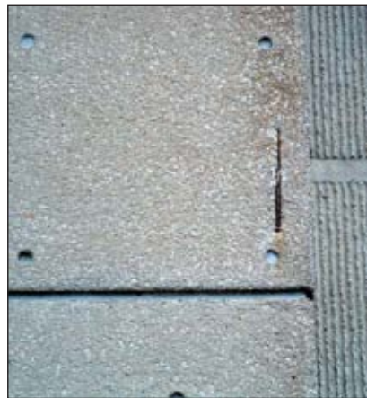
While minimum cover can be specified the cover that is ultimately achieved is frequently dependant on practical considerations.
