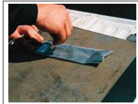
100 grams of Galvpatch being mixed for site repairs of hot dip galvanized steel
