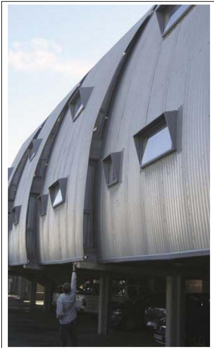
**“S” rib profiled coating class Z600 (SANS 3575) continuous hot dip galvanized sheeting was used as the material of choice in the stressed skin on the South Façade as well as for the roof sheeting on the North wing**
