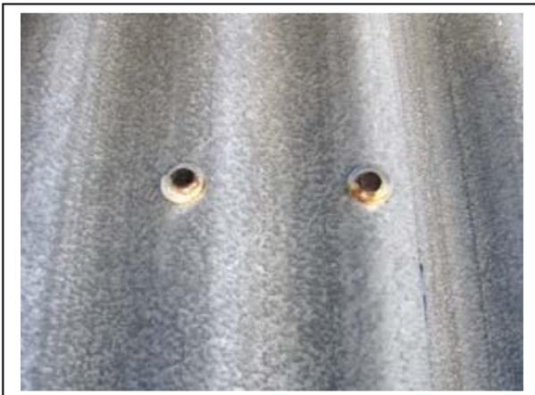
**A number of the original fasteners, which were unfortunately zinc electroplated, were showing signs of discolouration and rust**
