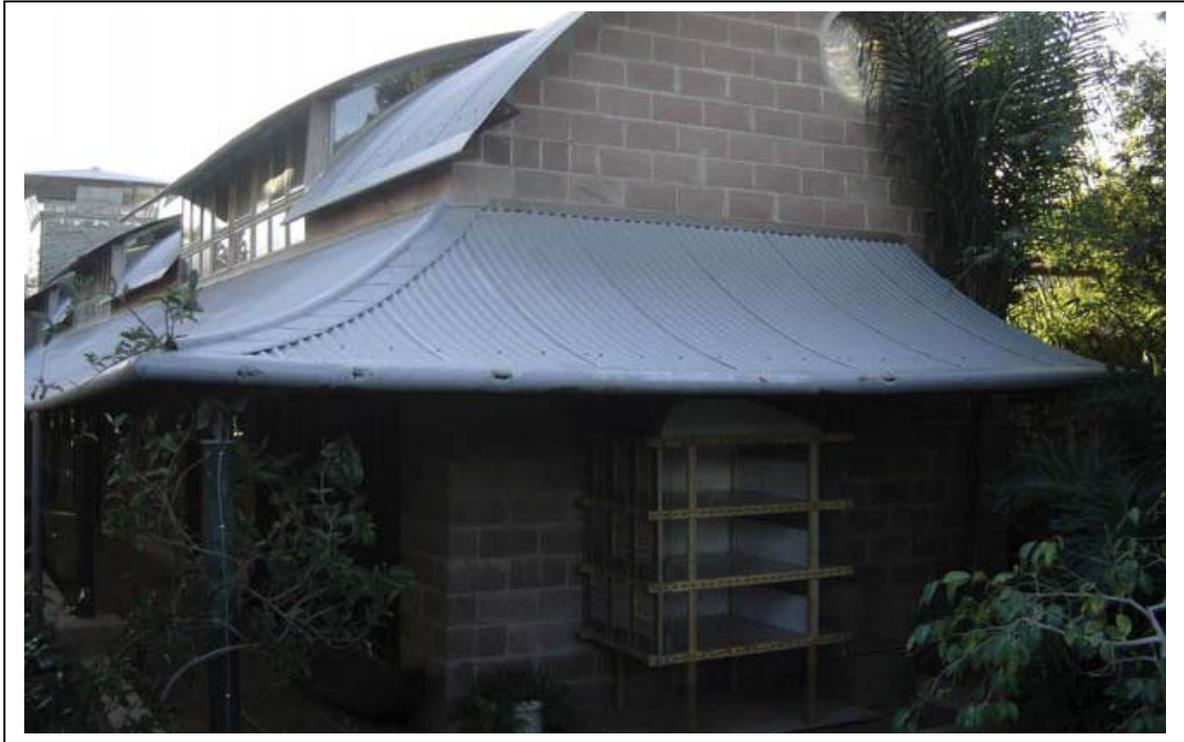
**This lip together with dust, debris and leaf deposits from the closest tree together with the normal rainfall, created the conditions for under deposit corrosion and the gutter over these 10 years corroded through in a few areas**
