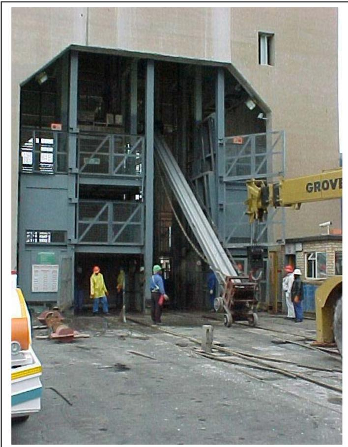
**Hot dip galvanized shaft guides being unslung onto the cage for transport down the mine for installation**
