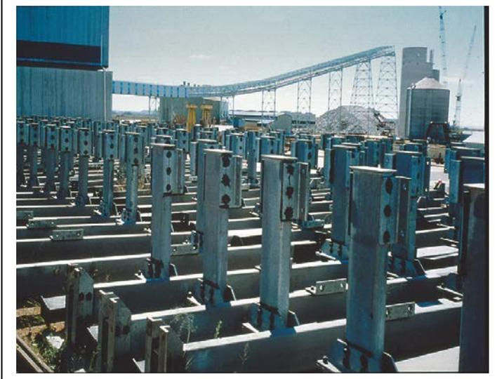
**Hot dip galvanized buntons with cold tar epoxy used to overcoat the fasteners and seal crevices**
