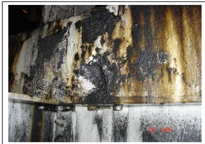
Two examples of the extent and severity of the corrosion conditions on painted steel
