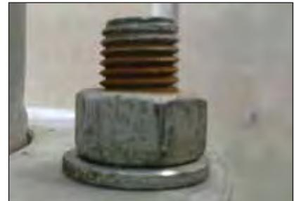
Photo 4: Corrosion products evident on a bolt thread after assembly. Causes could be re-tapping, or poor quality galvanizing both of which are unacceptable.
