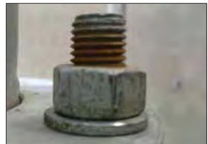
Photo 4: Corrosion products evident on a bolt thread after assembly. Causes could be re-tapping, or poor quality galvanizing both of which are unacceptable.
