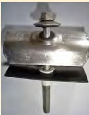
*If a stainless steel washer had been used there would have been no reaction between the Torspeed and the washer. We often find that contractors use aluminium washers rather than stainless steel washers as the aluminium washers are cheaper.*
