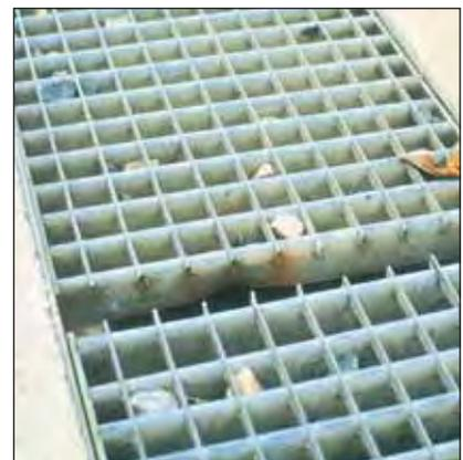
After 26 years of mild marine exposure, this site cut unrepaired hot dip galvanized steel grating still offers cathodic protection at the cut ends.
