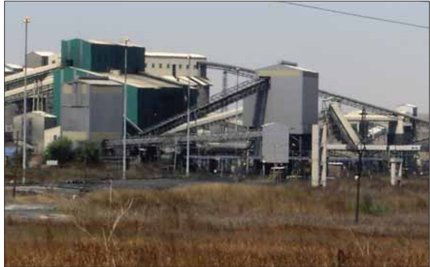
General view of Douglas Colliery.
