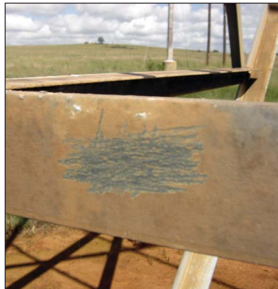
Site No 1. – After removing the “apparent” rust discoloration, the underlying hot dip galvanized coating measured 65,4µm. Accuracy of the instrument is approximately 5%.
