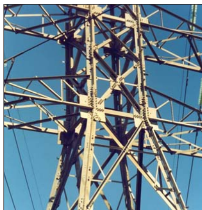
Site No 3. General condition of the tower after 25 years of service. A subsequent paint coating (providing a duplex coating system), has been recommended in order to extend the life of the structure.
