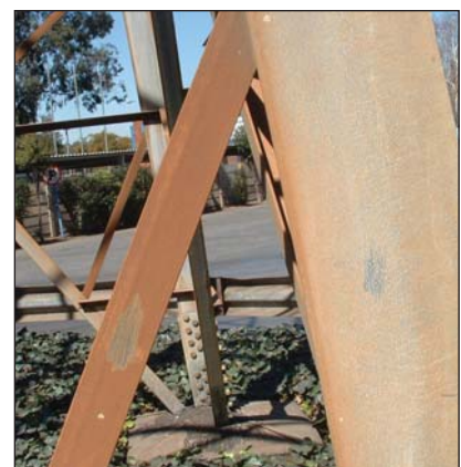
Site No 2. After the removal of the discoloration, i.e. corrosion products, the hot dip galvanized coating thickness measured to be 119µm.
