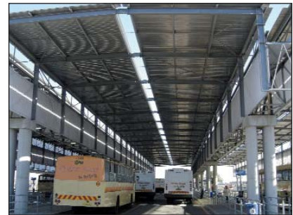
An end view of one of the bus shelters which forms part of the new Transport Interchange.
