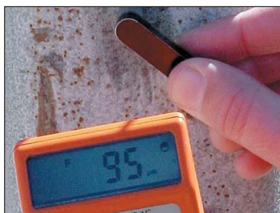
Coating thickness (95µm) on the scraped surface.
