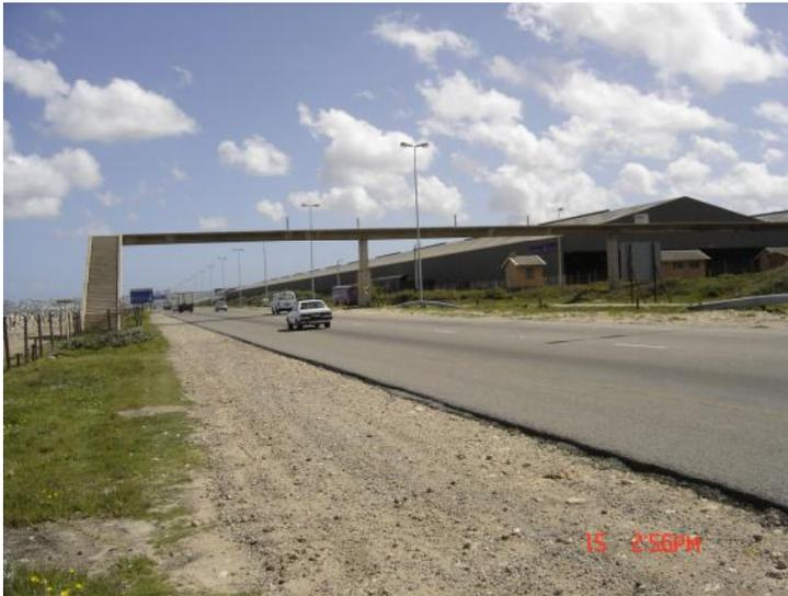
The site of the 40-year-old pedestrian bridge (No B776), due to be demolished. (April 2005). It was established that hot dip galvanized reinforcement was used in the approach stairway, which was on the sea facing side, indicated on the left of the photograph, with the sea some 50 meters further left.
