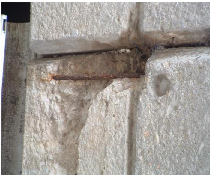
Corroded reinforcement resulting in the "spalling off" of the concrete. Note the lack of concrete cover.
