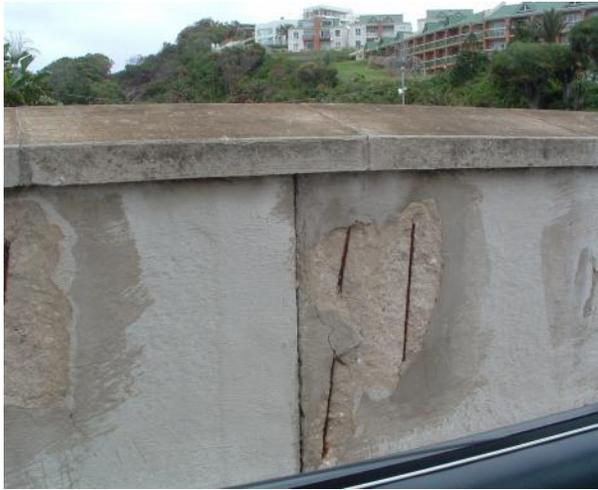
Repairs to the concrete on this bridge structure proved to be unsuccessful in that the corroding reinforcing bars have again removed the concrete.
