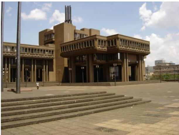
Johannesburg Civic Centre is an example of hot dip galvanized reinforcement being used as an architectural requirement to prevent rust staining on the slender (low concrete cover) fascia panels. Original construction period was from 1964 through to 1968. A recent inspection no sign of rust staining was evident.
