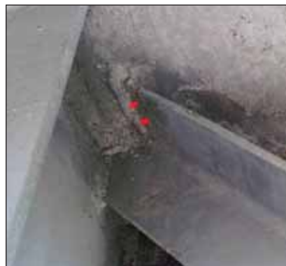
Figure 1b: The image on the left shows the connection between the angle section chord and the two I-beam chords at a 90° T-joint. The arrows indicate the position of a crack in the angle section chord. The image on the right shows the same crack. The crack had developed in the unaffected base metal next to the weld heat affected zone of a fillet weld.
