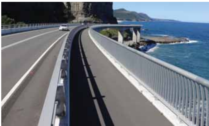
New South Wales sea cliff bridge with single car lanes and adjacent pedestrian walkway. All barriers and rails hot dip galvanized.
