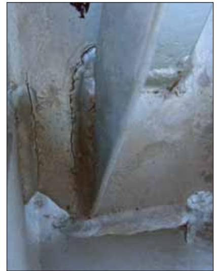
Figure 2c: Examples of cracks in the web of a transverse I-beam chord at fillet welds at the connection between a diagonal angle section chord and transverse I-beam chord in the top image in Figure 2a. The cracks had developed at highly restrained welds.
