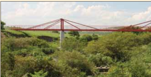
Zwelitsha Pedestrian Bridge over the Buffalo River, Eastern Cape – hot dip galvanized and painted.
