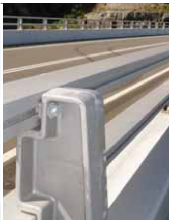
Well-designed bracket for attachment of guard rails on the NSW cliff bridge.
