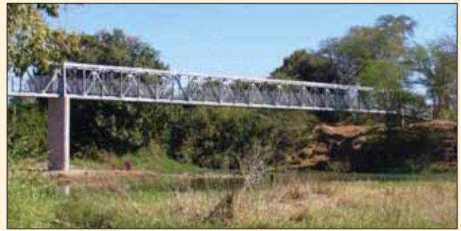
Makanise Bridge known as Pongola Bridge, KwaZulu Natal Richards Bay area.
