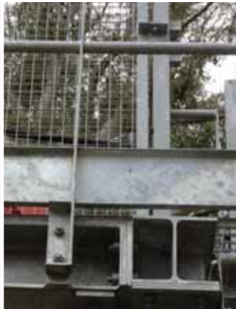
Scenic World, Blue Mountains, Australia. The entire cable car docking station, walkways, handrails and fence paneling has been hot dip galvanized.
