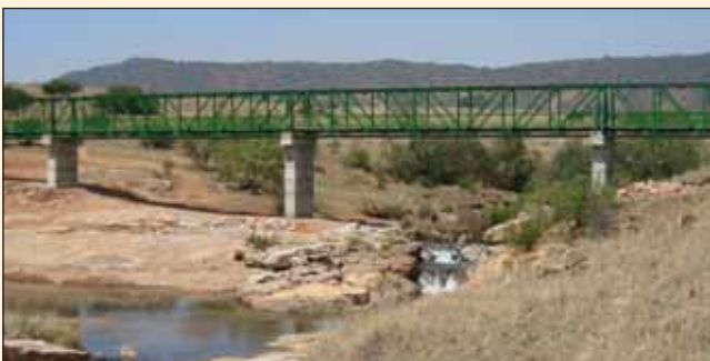
Ntombe River Bridge, Northern KwaZulu Natal near the site of the Battle of Ntombe drift 1879 – hot dip galvanized and painted.
