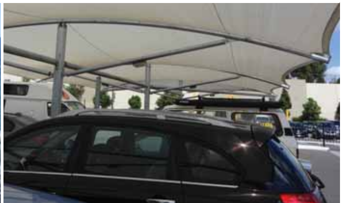
The support structures for car ports.
