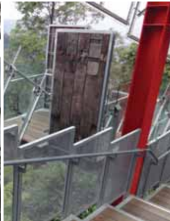
Scenic world again, illustrating the architects use of the natural elements of steel and wood and the contrasting use of duplexing-paint on galvanizing – to achieve the desired aesthetic effects.
