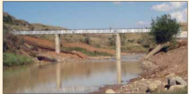
Insuze Bridge – KwaZulu Natal.
