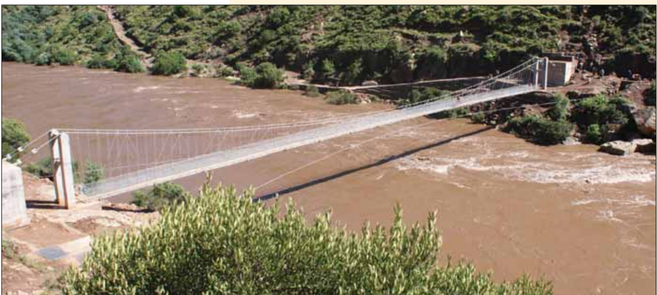
Bisi Pedestrian Bridge, KwaZulu Natal Umzimkhulu.
