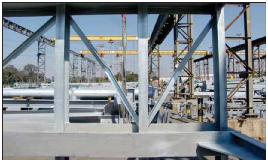
Figure 2d: Examples of distorted/buckled angle section chords. The cracks were associated with the welded connections between these diagonal angle section chords and the webs of the transverse I-beam chords.
