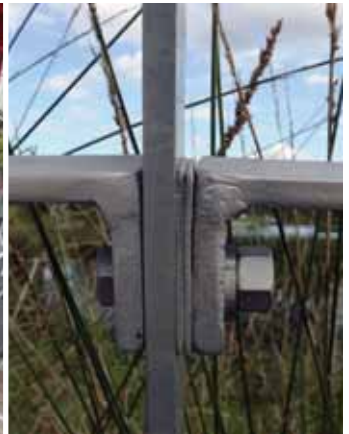
A very standard hand rail system, but note the engineering attention to detail. The holes are slotted during manufacturing to avoid on site modifications and all the spacing shims are galvanized. These design considerations eliminate the risk of compromised corrosion control.
