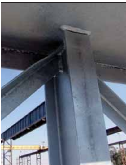
Figure 2d: Examples of distorted/buckled angle section chords. The cracks were associated with the welded connections between these diagonal angle section chords and the webs of the transverse I-beam chords.
