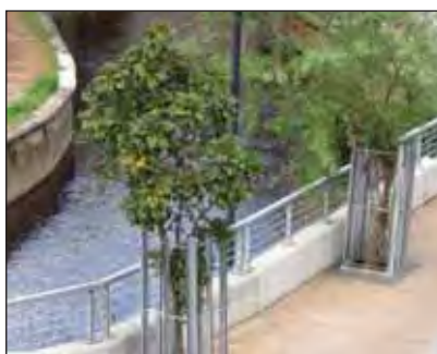
The hot dip galvanized handrails and tree supports provide an edge to the river way, reducing the possibilities of vagrants.
