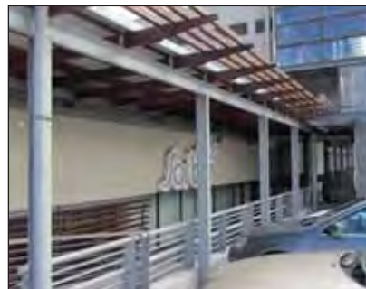
The combination of dark timber and hot dip galvanized steel provided an aesthetical appeal to some of the pergolas in the parking bays.
