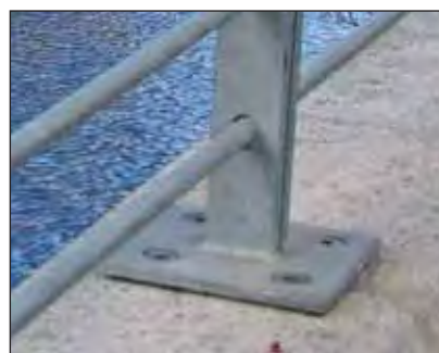
In order to create a neat, flush finish that enhanced the overall design hot dip galvanized sleeve anchors were used with countersunk studs.
