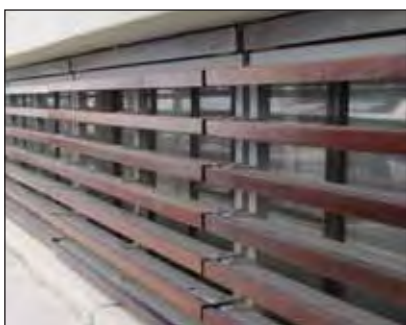
Dark timber facades were attached to inaccessible hot dip galvanized steelwork.
