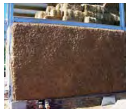
One of the exterior walls showing the "scratch coat" which is applied using hands and wooden sticks.
