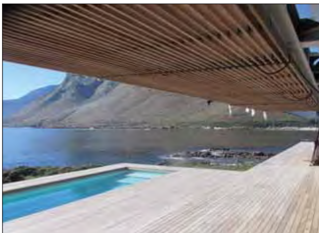
View from the timber deck with the hydraulically operated slatted timber shutters in their open position.
