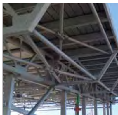
The view on the hot dip galvanized steel gable end installation.
