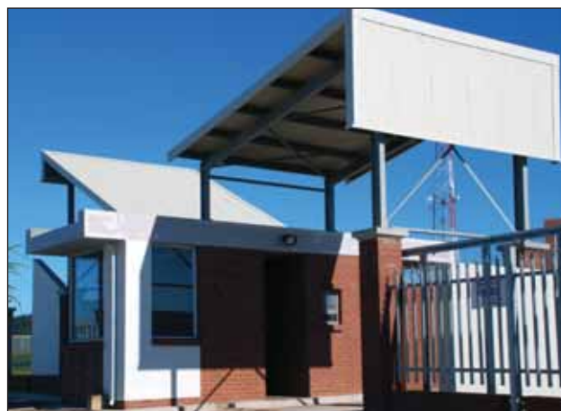
Gate house and hot dip galvanized steel canopy.
