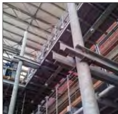
The interior walkway installation comprises natural hot dip galvanized steel.
