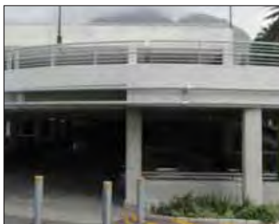
Modular design and fabricated hand rails were successfully hot dip galvanized with very little site alterations and unnecessary coating repair.
