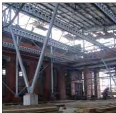
Early view of the hot dip galvanized support steelwork for the call centre mezzanine.
