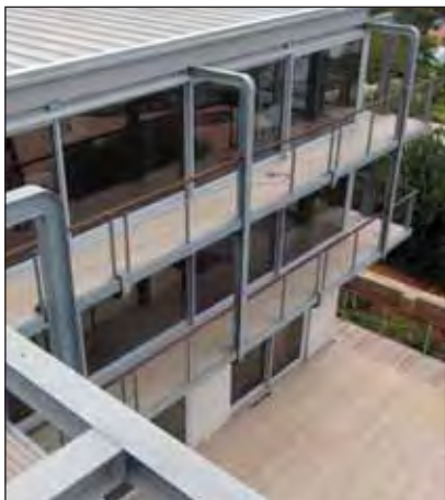
The hot dip galvanized framing clearly defines the extremities of the timber floor decking and the glazing components.
