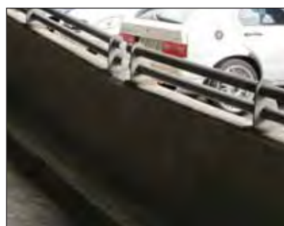
Modular design and fabricated hand rails were successfully hot dip galvanized with very little site alterations and unnecessary coating repair.
