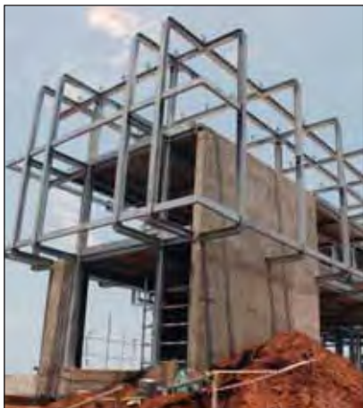
The hot dip galvanized steel frame forms a rigid support onto which the flooring, glazing and floor decking is hung.
