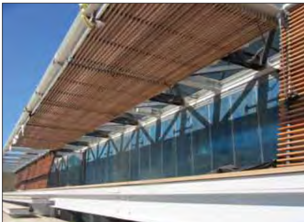
Another view showing the hydraulically operated slatted timber shutters in their open and semi-closed positions.
