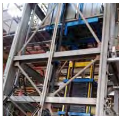
The hot dip galvanized steel lift installation.
