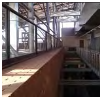
The smoke extraction installation showing interior hot dip galvanized steelwork.
