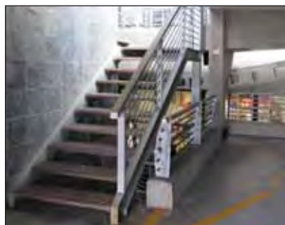
All vertical circulation, staircases between parking decks, are hot dip galvanized for minimum maintenance.
