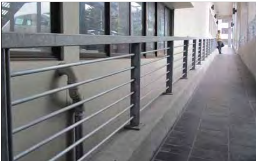
All horizontal and vertical handrails are hot dip galvanized to minimise maintenance.
