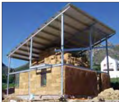
Infill straw bale walls are fully supported by the hot dip galvanized portal frame.
