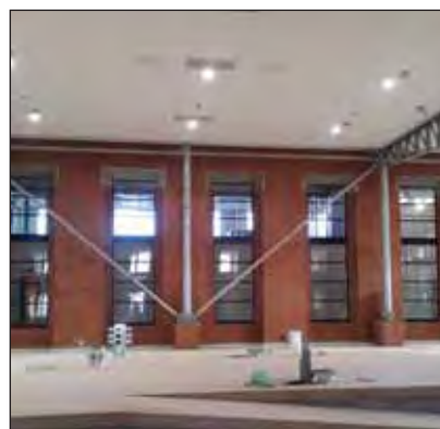
The call centre ceiling installation showing the exposed hot dip galvanized steelwork.
