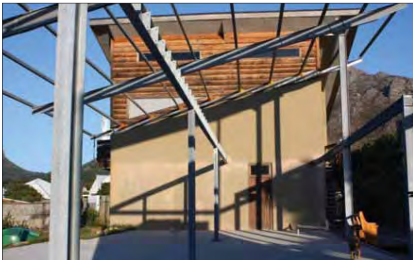
A view on the hot dip galvanized steel portal frame as it projects from the initial phase of the building.
