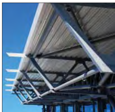
Completion of the hot dip galvanized steelwork at the western gable end.
