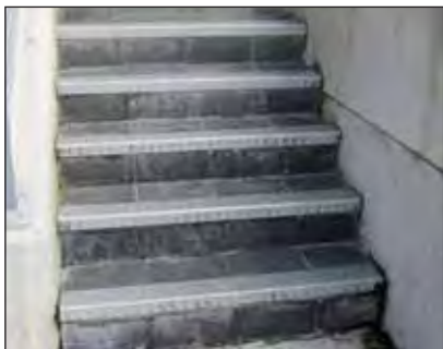
Hot dip galvanized steel stair nosings were used on the leading edges of tiled stair treads and risers.
