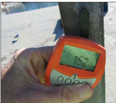
Zinc chloride salts removed and the residual coating thickness measured - 152 \mu m.
