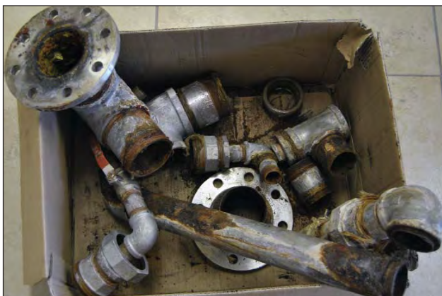
Photo 1: Some of the corroded products after being removed and replaced with copper pipes.
