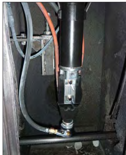
Electric drive arc spray gun spraying zinc onto the welded area.
