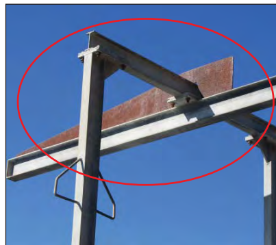
Photos above show the gantry with some uncoated carbon steel that has been added. This will in time tend to discolour the hot dip galvanizing when the former begins to rust. Photo right shows the inappropriately coated fasteners, which were most probably originally only zinc electroplated, requiring replacement or coating repair.
