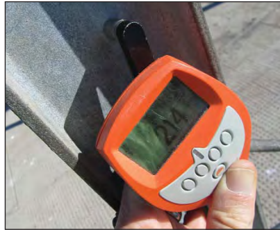
Zinc chlorides salts almost non-existent due to the orientation of the web wrt the direction of the prevailing wind, coating thickness - 214 \mu m.
