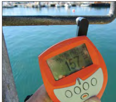
Zinc chlorides salts almost non-existent on round bar climbing hoops, coating thickness - 157 \mu m.
