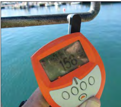
Zinc chlorides salts almost non-existent on round bar climbing hoops, coating thickness - 158 \mu m.
