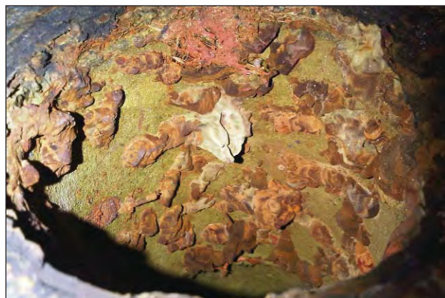
Photo 2: Tubercles found inside the pipes.
