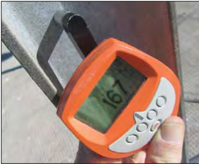
Zinc chlorides salts almost non-existent due to the orientation of the web wrt the direction of the prevailing wind, coating thickness - 167 \mu m.
