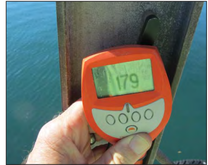
Zinc chlorides salts almost non-existent due to the orientation of the web wrt the direction of the prevailing wind, coating thickness - 179 \mu m.
