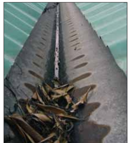
Leaves and debris in a gutter can have a marked effect on the service life.
