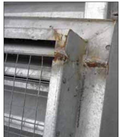
Photo above left shows the sound baffle with rusted expanded metal after 2 - 3 months exposure. Photo above right shows the necessary repair required after manufacture of the outer louvres.
