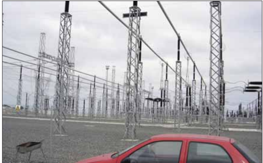
General view of the steel masts at the plant. It is generally accepted that all steel that is used to manufacture components for power plants and power conveyance pylons are at least hot dip galvanized to SANS 121 for corrosion protection.
