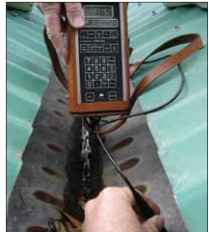
Coating thickness in the gutter, 16.5 micrometres.
