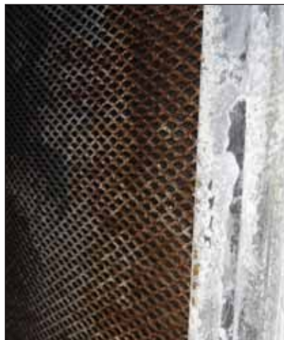
Photo above left shows the sound baffle with rusted expanded metal after 2 - 3 months exposure. Photo above right shows the necessary repair required after manufacture of the outer louvres.
