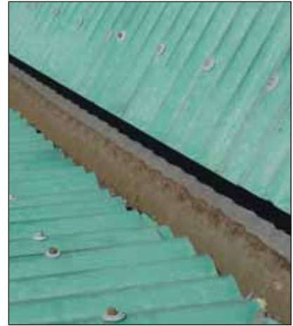
Corrosion of the pre-galv material has taken place due also to the frequent blocking of the gutter downpipes.
