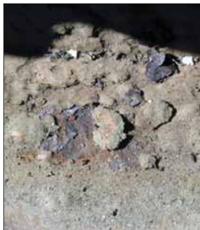
The inside of the gutter in certain areas was in an advanced state of corrosion.
