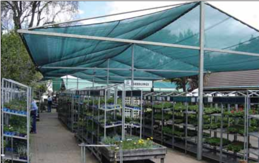
All the structures and utility steelwork at Starck Ayers is hot dip galvanized, a fitting compliment to the hot dip galvanizing industry.
