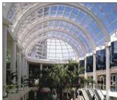
Australian Plaza, near the Pacific beach, with purlins and glazing frames protected by a duplex system based on polyurethane.
