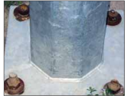
Photo 10: Make use of hot dip galvanized holding down bolts for long term maintenance free life.
