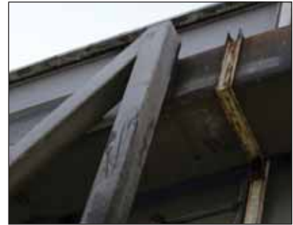
After years of exposure the performance of the painted bracketry that was added to the original buffer sign gantry can be visually compared to the hot dip galvanized coating.
