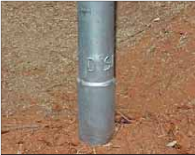
Photo 8: Differential aeration may be prevented by an additional steel sleeve situated above and below the ground level.
