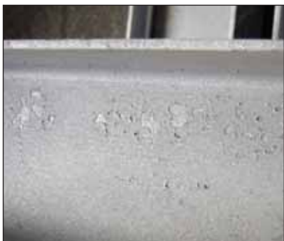
General view of the damaged hot dip galvanized coating on the web of the structural section.
