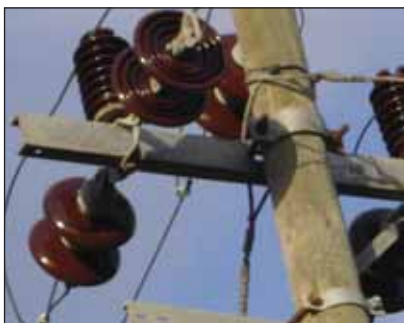
Photo 2: Outreach arms are usually hot dip galvanized steel. Care should be taken that fasteners also be hot dip galvanized for long term corrosion control.
