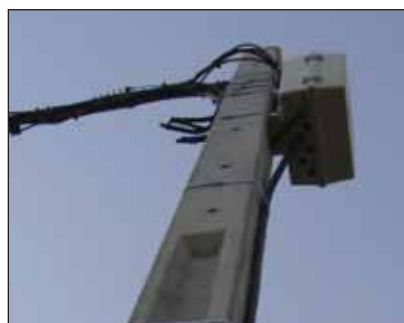
Photo 7: Concrete poles often need outside junction boxes to accommodate incoming cables.
