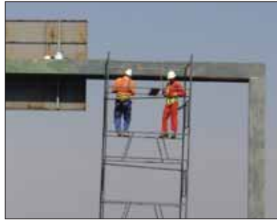
Repainting of insitu sign gantries for a successful maintenance free coating is dangerous and extremely difficult to achieve.
