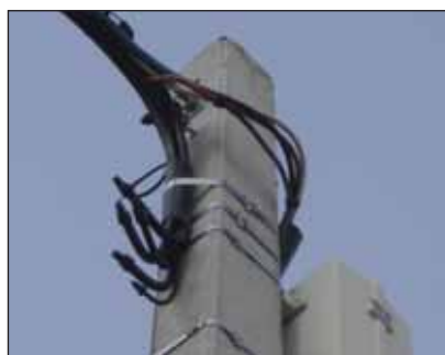
Photo 6: Cables are attached to the outside faces of the concrete pole, limiting its aesthetical appeal.
