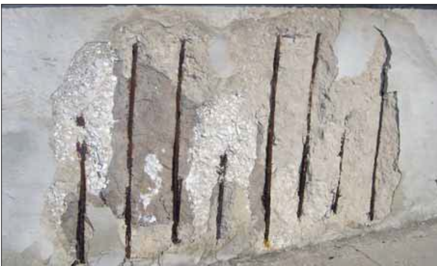
Spalling concrete indicates a potential for structural failure. Once spalling has occurred, it becomes very difficult and expensive to repair.
