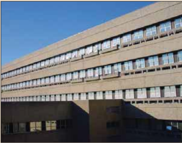
New Grootes Schuur Hospital, Cape Town.
