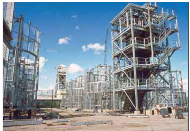
Typical example of hot dip galvanized shaft station steel structure, beginning check assembled followed by dis-assembly to be transported underground to be re-erected.
