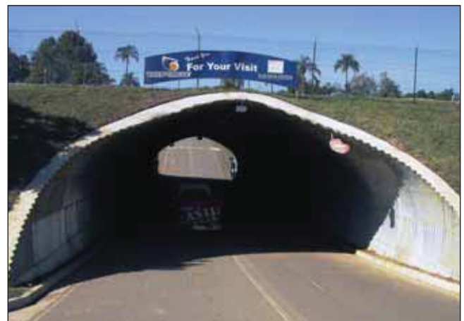
Armco Superspan arch as an underpass on the horse race track.
