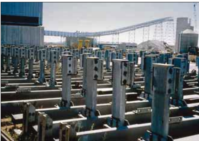
Hot dip galvanized cross shaft steel "Buntons" used together with the shaft guides to equip the shaft on a gold mine.
