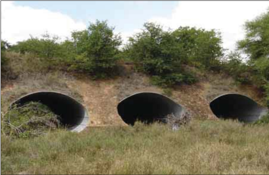
Two examples of hot dip galvanized steel structures buried in soil. In both cases a neutral backfill (less corrosive) is the first step of providing an envelope around the structure as part of combating soil side corrosion.
