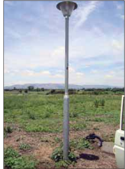
Two examples of hot dip galvanized steel structures buried in soil. In both cases a neutral backfill (less corrosive) is the first step of providing an envelope around the structure as part of combating soil side corrosion.
