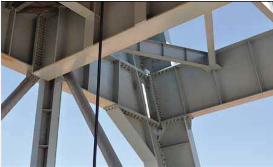
Bolted connection at Bakubung Platinum Mine Headgear.
