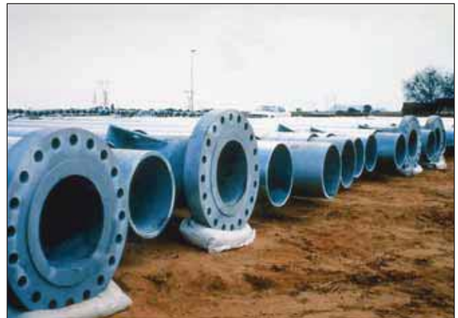
Hot dip galvanized high pressure service pipes waiting to be moved underground.
