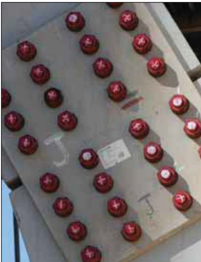
Quality checks on a connection.
