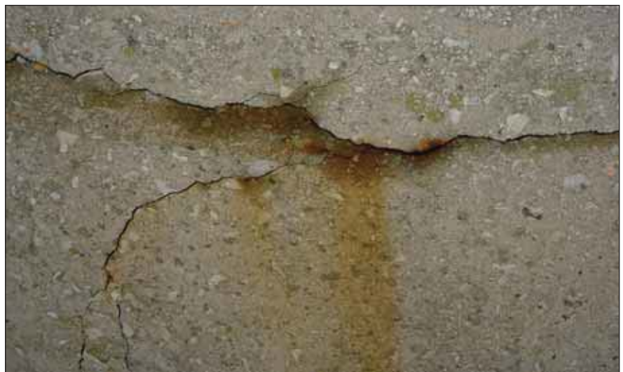
Ingress of corrosive substances is first indicated on the concrete surface by rust stains, followed by cracks.
