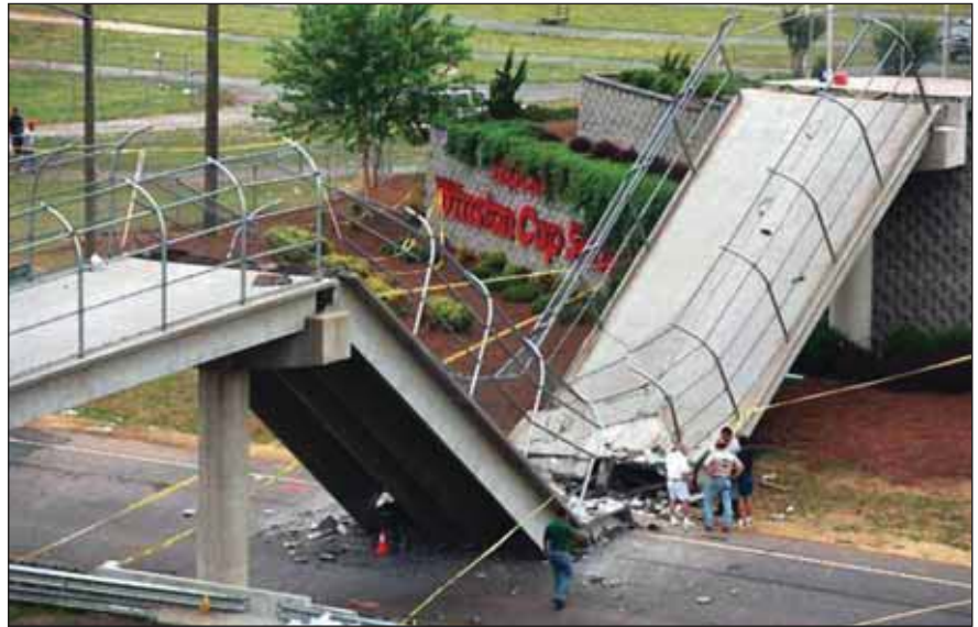
Catastrophic structural failure example, attributed to corrosion of reinforcement.
