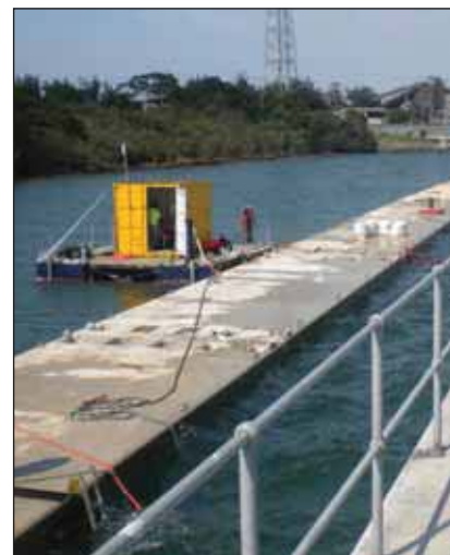
The pontoons in their final position alongside Berth 208.
