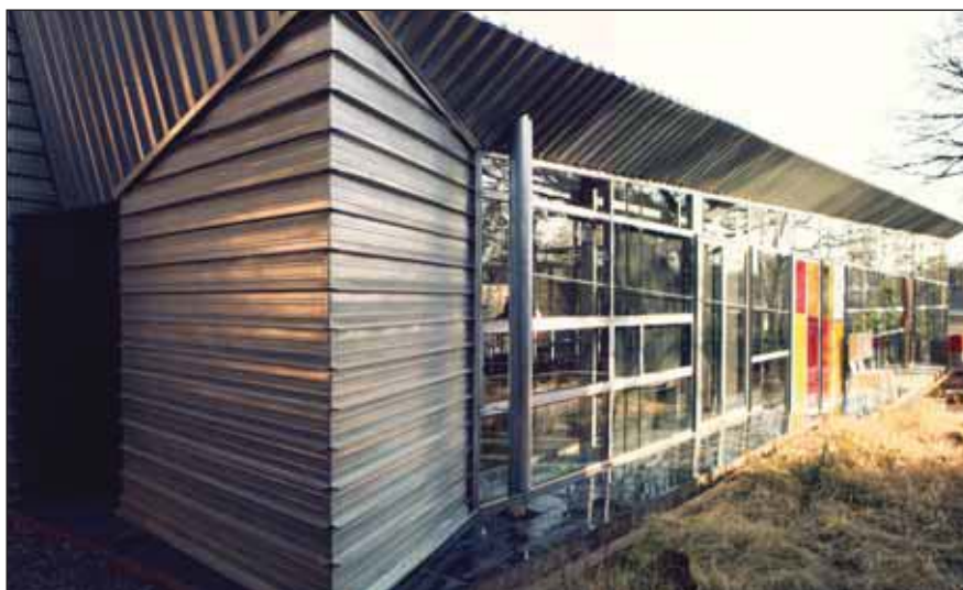
The total steelwork structure with glass windows and sheeting clad gable end was custom fabricated to the client's specifications. The project is a showcase of innovation, technology and the creative use of hot dip galvanized steel.
