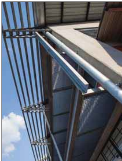
High level 3m wide cantilever hot dip galvanized steel truss, supports galvanized sun control grids below it.
