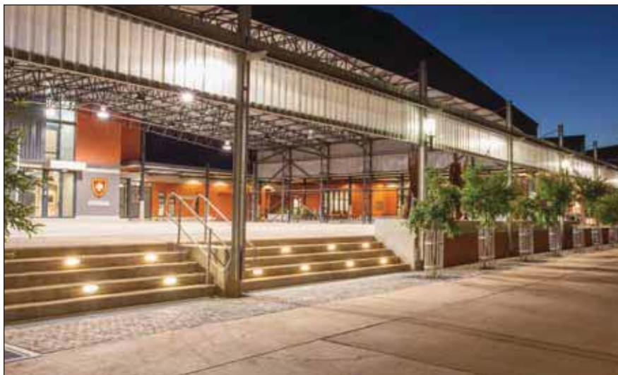
The use of a hot dip galvanized steel finish for the external elements impacts positively on the long term sustainability of the project.
