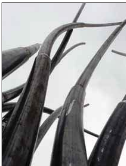
Checking the final configuration of the pole artwork before hot dip galvanizing.
