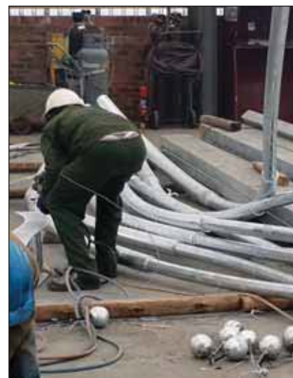
After hot dip galvanizing, adding the final touch up with zinc metal spraying prior to painting.
