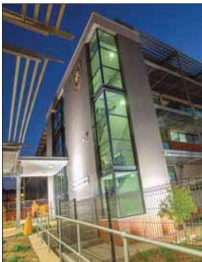
Hot dip galvanized steel canopies provide protection for the pedestrian walkways linking different buildings across the site.
