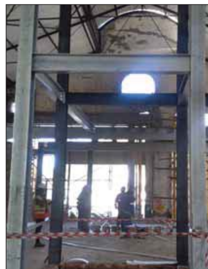
A view of the internal duplexed steelwork during construction.
