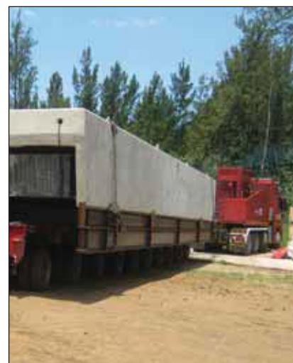
A completed pontoon arriving at the beach by horse and trailer.
