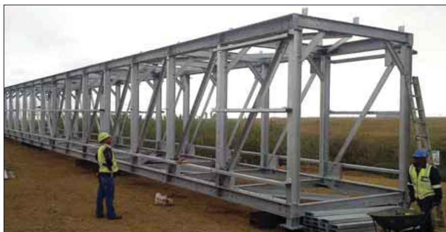
The completely assembled hot dip galvanized bridge.
