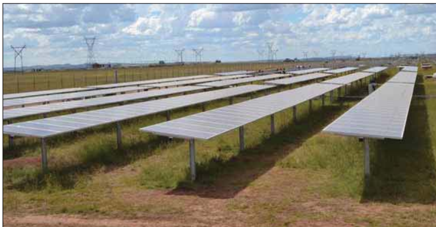
The unique feature of the Contour Track system is that it can be adapted for any terrain type. This eliminates the need for major earthworks resulting in a structure that has minimal impact on the surrounding environment.
