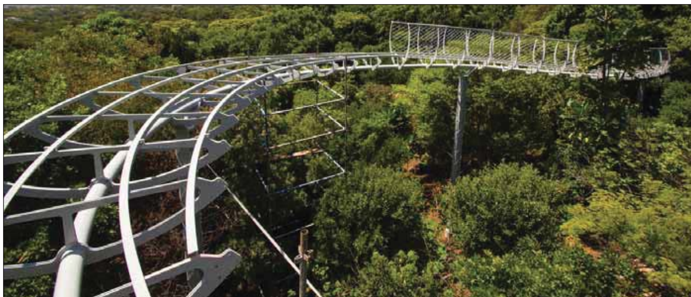
The partially finished "Boomslang" winds and dips its way through and over trees of the Arboretum.
