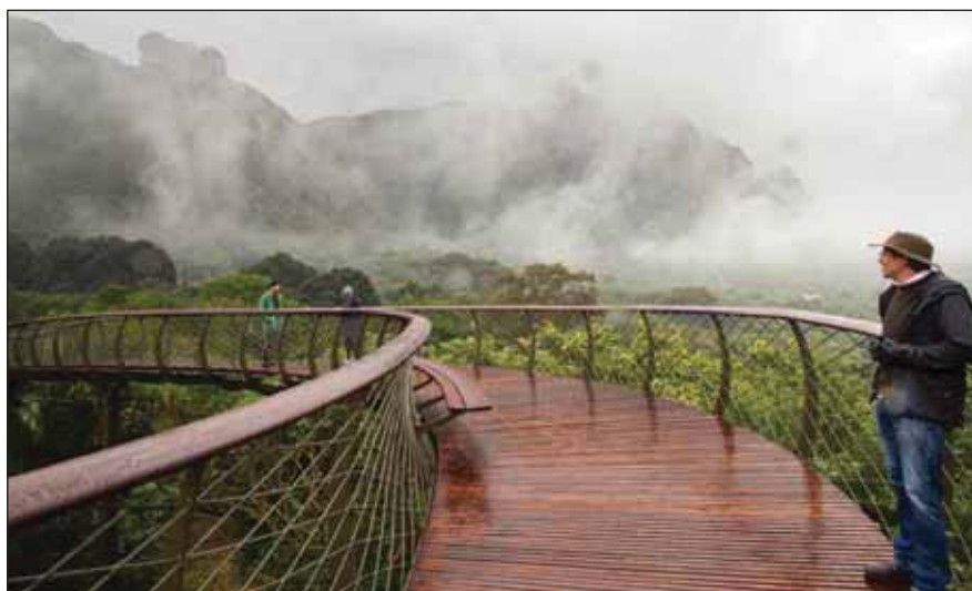
While the walkway has been designed to move as a snake would, it is intrinsically safe and can accommodate up to 1 300 people at one time.
