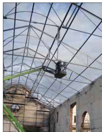
The roof rafters which were replaced following a fire in the nineties by a similar duplex coating system, were reused.
