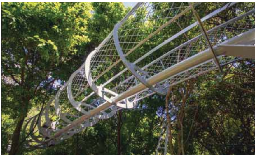
The carefully duplexed sections were hoisted by crane on site using soft slings and bolted in position to minimize disruption to the trees during construction.
