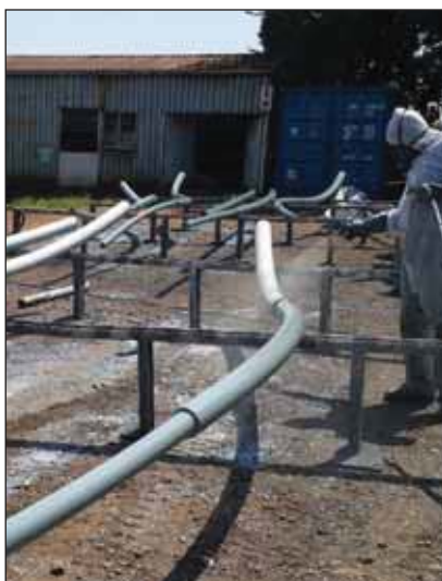
Poles being primed with the first coat of paint.
