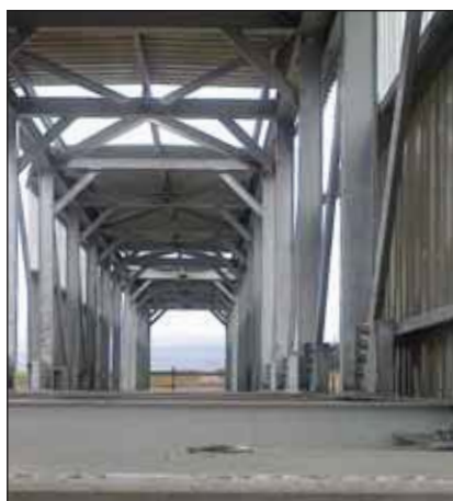
A view of the bridge through the centre.
