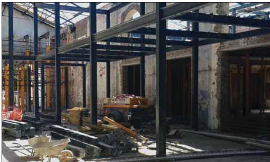
A view of the internal duplexed steelwork during construction.
