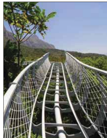
The carefully duplexed sections were hoisted by crane on site using soft slings and bolted in position to minimize disruption to the trees during construction.
