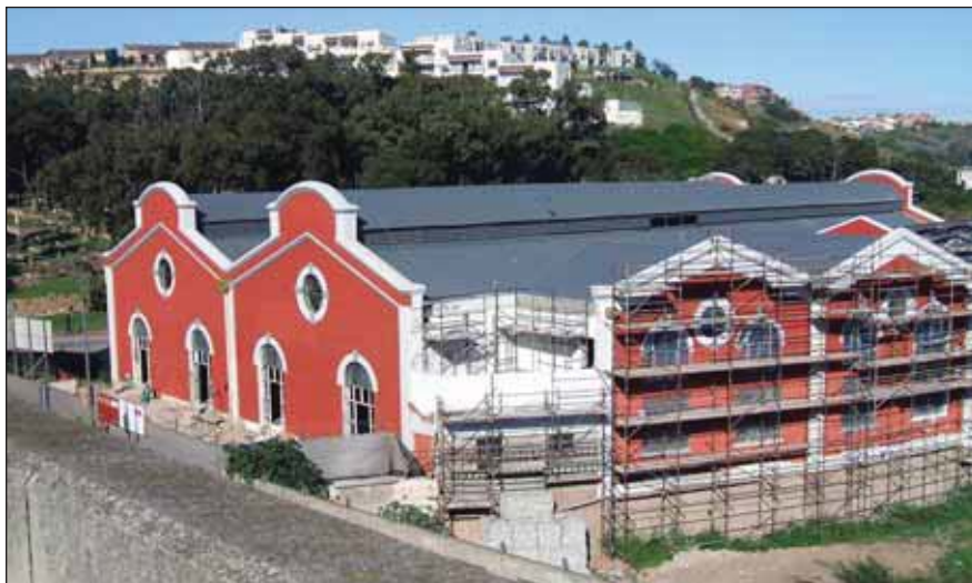
The revamped Tramways Building nearing completion.
