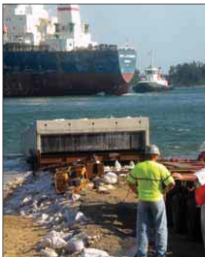
A pontoon being launched into the sea being towed to its final location.
