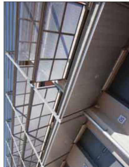
High level 3m wide cantilever hot dip galvanized steel truss, supports galvanized sun control grids below it.
