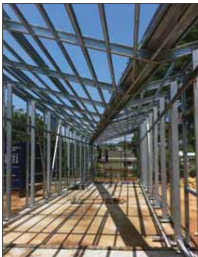
The steelwork structure comprises mainly of galvanized steel hollow sections forming the columns and window frames and galvanized hot rolled sections forming the rafters and eaves beams.
