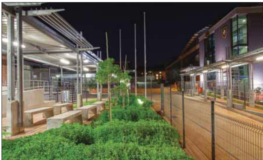
Hot dip galvanized steel canopies provide protection for the pedestrian walkways linking different buildings across the site.
