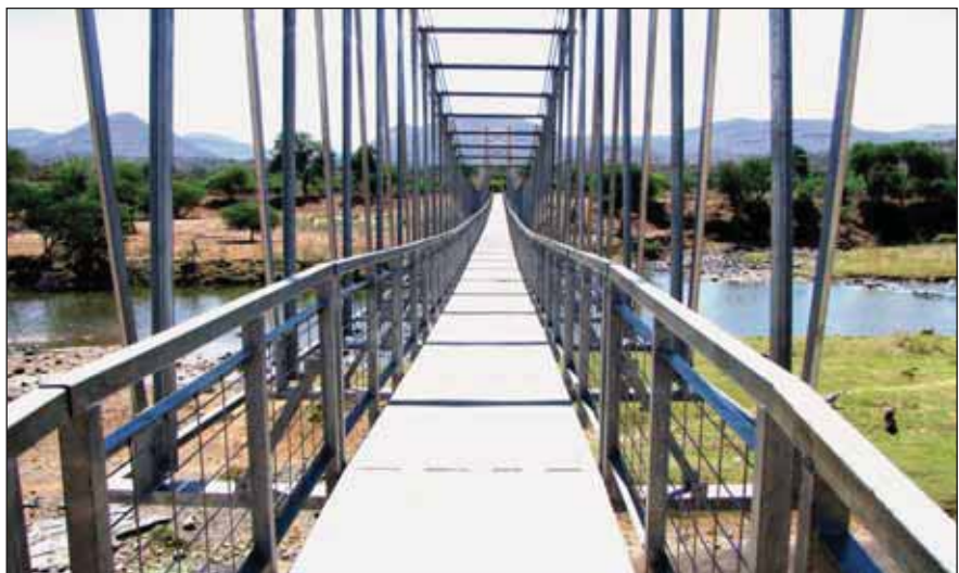
The hot dip galvanized suspended girder type walkway and components are fixed to two support cables that are fixed 120m apart on either side of the river.
