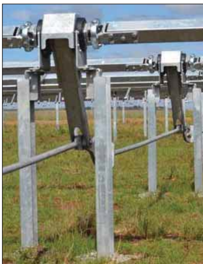
Hot dip galvanizing has over the decades proved to be an effective corrosion protection system for solar projects.
