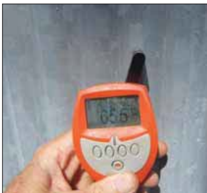
A typical coating thickness reading (65.6um) on a radiator fin after many years of exposure. See recent Case Histories.
