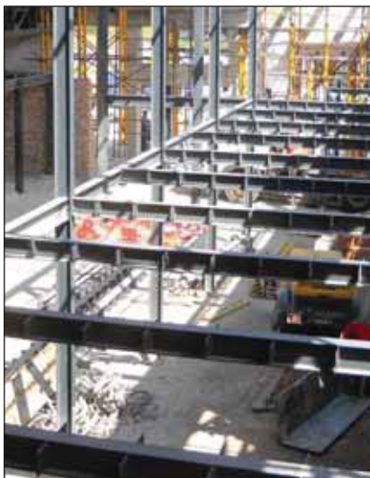
Further views of the new duplex coated steelwork installed to support the new mezzanine floor.
