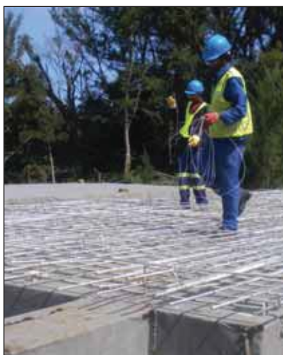
The coated polystyrene block configuration with the initial layer of hot dip galvanized reinforcing bars prior to casting the concrete.
