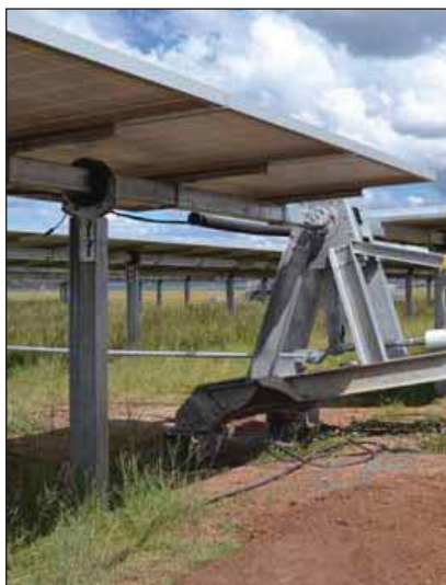
These frames allow the standard solar panels to rotate up to 90°, exposing them to UV rays from sunrise to sun set.
