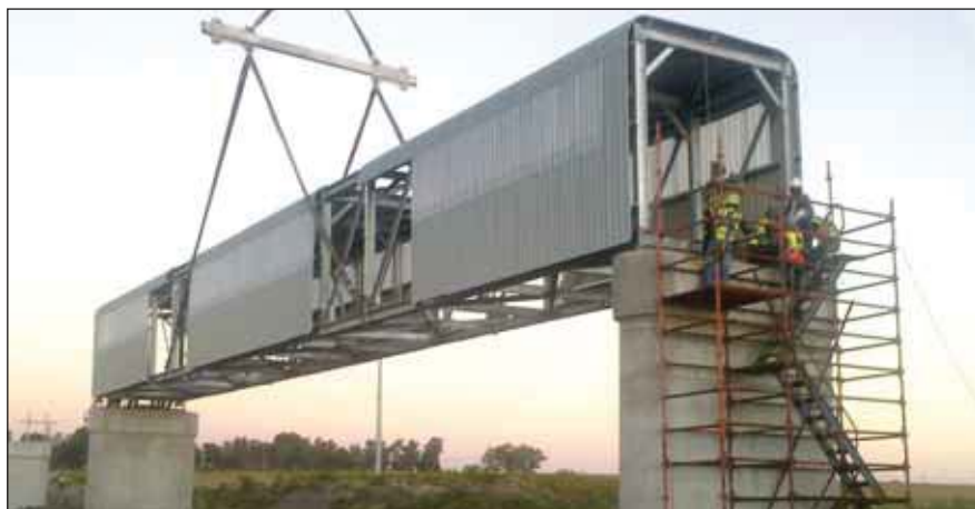
The hot dip galvanized bridge together with side and top cladding hoisted into position over the river.
