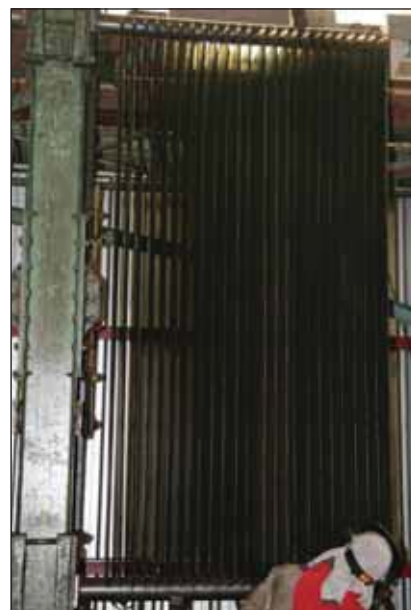
Completing the manufactured radiator.
