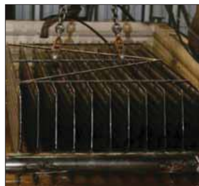
Pressure testing the completed radiator to ensure no leaks.
