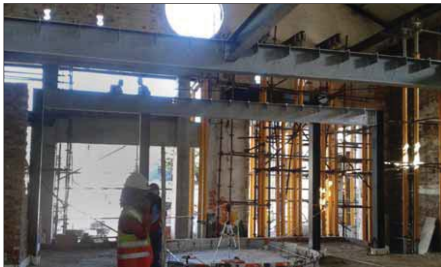
Further views of the new duplex coated steelwork installed to support the new mezzanine floor.
